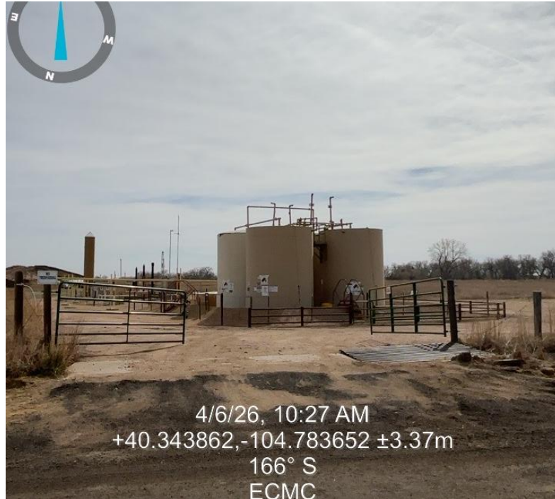
Location Entrance from 396
