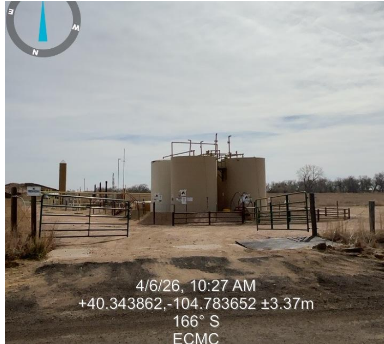
Location Entrance from 396
