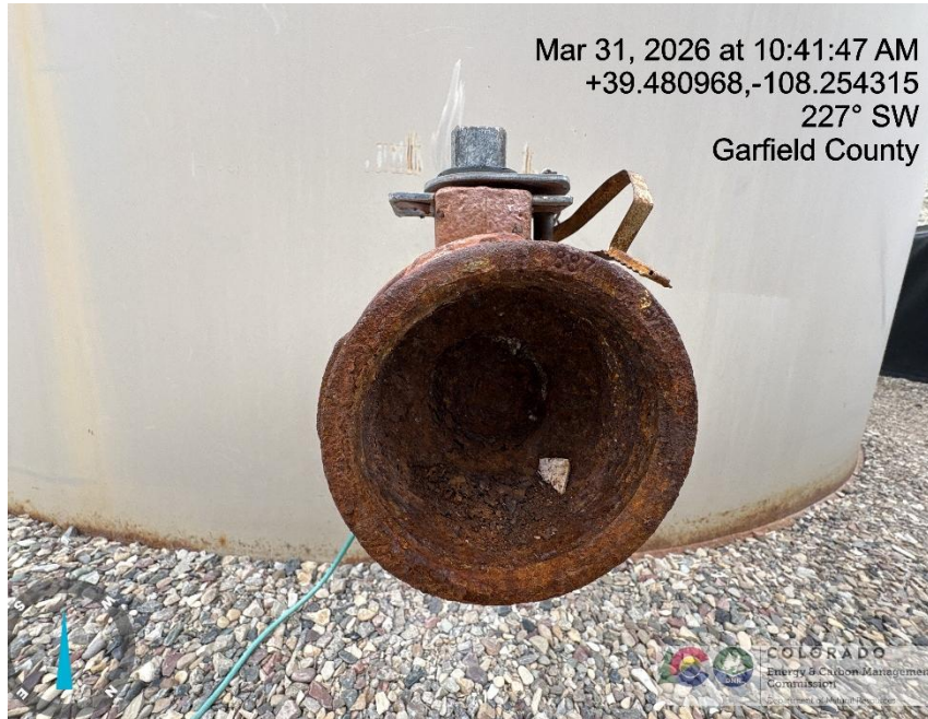
Photo # 3971 Open ended load line
