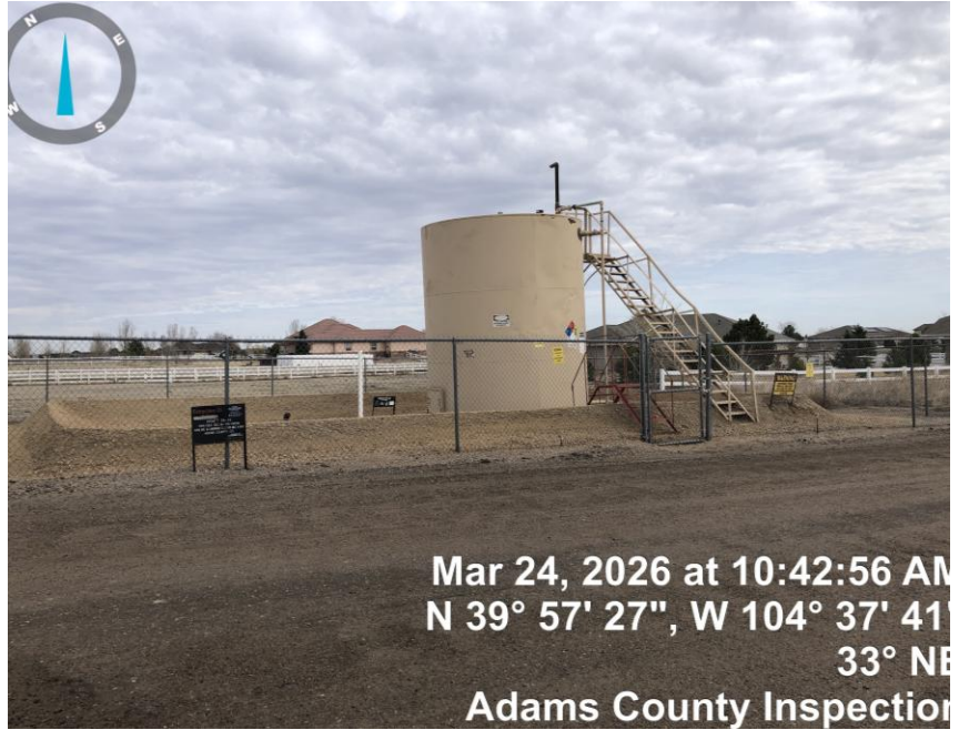
PHOTO#2 PRODCUTION TANKS
