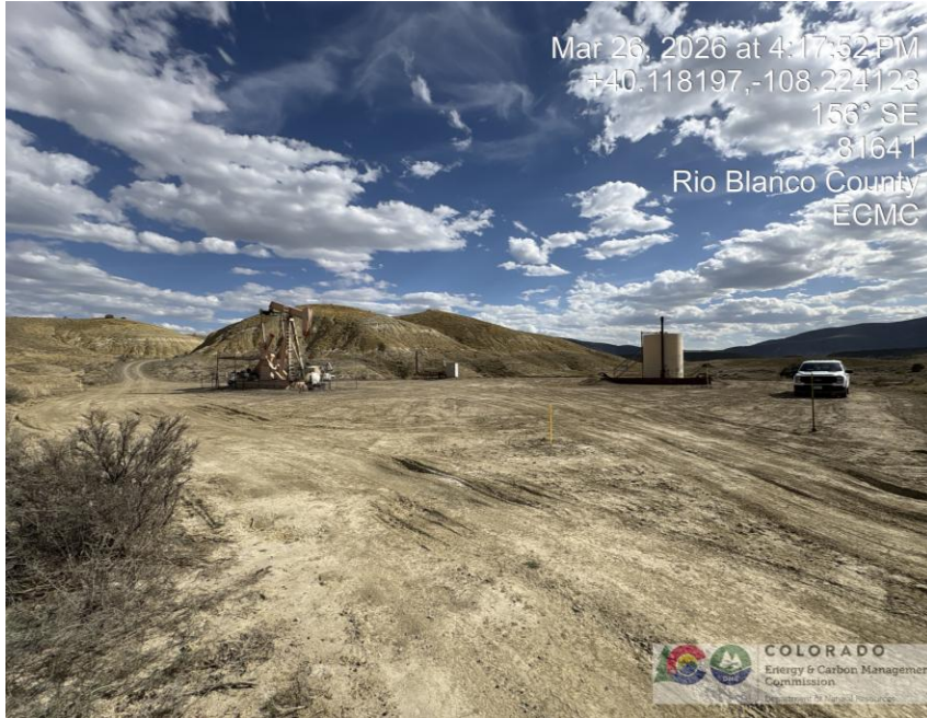
Photo # 3996 NW corner of location
