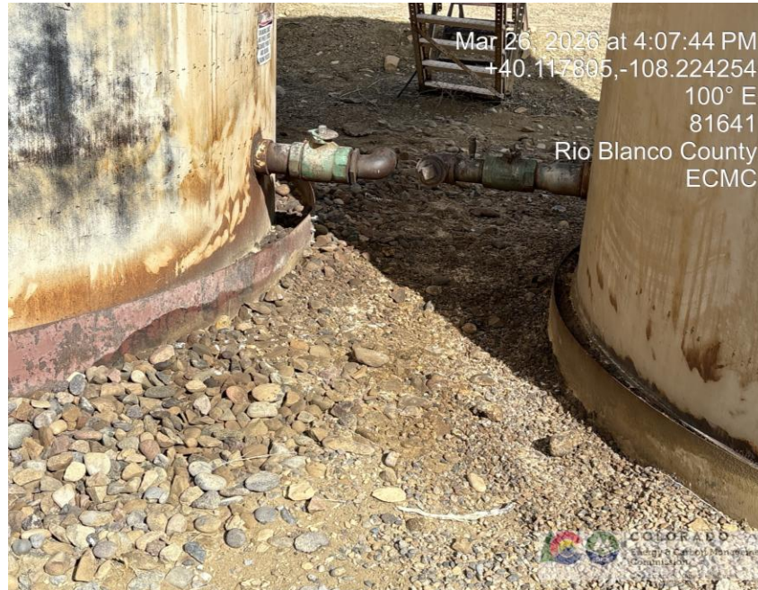
Photo # 3991 Stained soil
