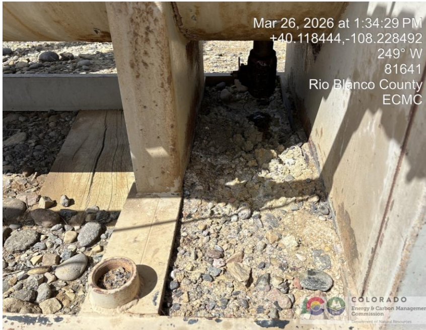
Photo # 3877 Stained soil beneath treater
