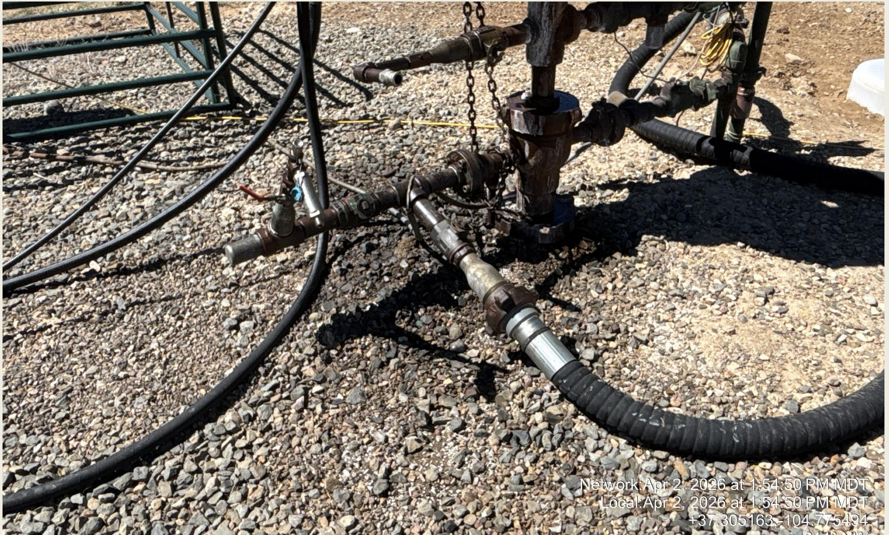
PHOTO 5: AREA OF IMPACTED SOIL AROUND WELLHEAD. Conduct maintenance on equipment, cleanup stained material and review self inspection processes. COMPLY WITH RULE 1002,(2).D. THIS IS THE 3 RD NOTICE FOR THIS CA. IT APPEARS THAT THE OTHER AREAS OF IMPACTED SOILS AROUND LOCATION HAVE BEEN ADDRESSED HOWEVER AROUND THE WELLHEAD IS GETTING WORSE THE LEAK MUST BE ADDRESSED IMMEDIATE ACTION IS REQUIRED.
