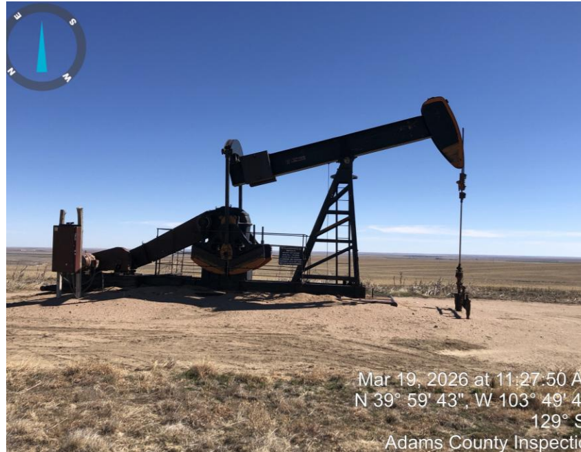
Photo #1 Pump jack.
