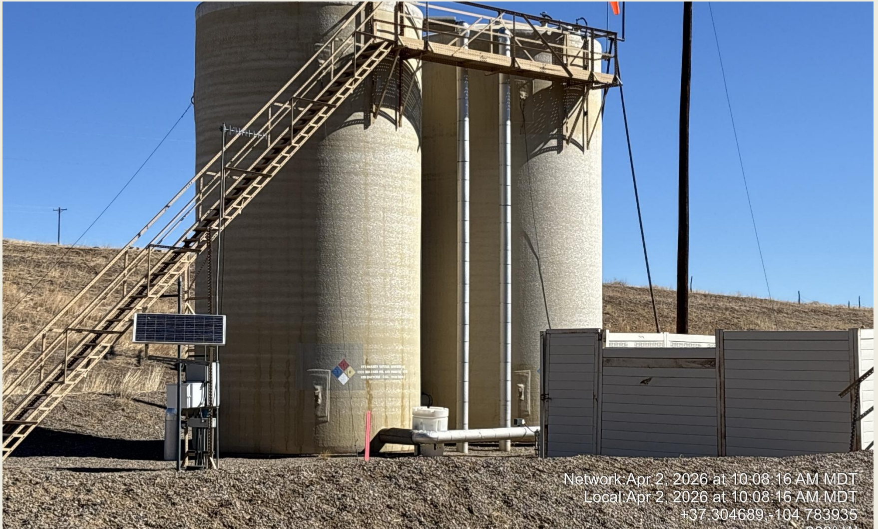
PHOTO 5: SIGN WITH ALL WELLS SERVICED BY TANK BATTERY NOT POSTED. POST SIGN PER RULE 605e. CA DATE 5/2/2026.
