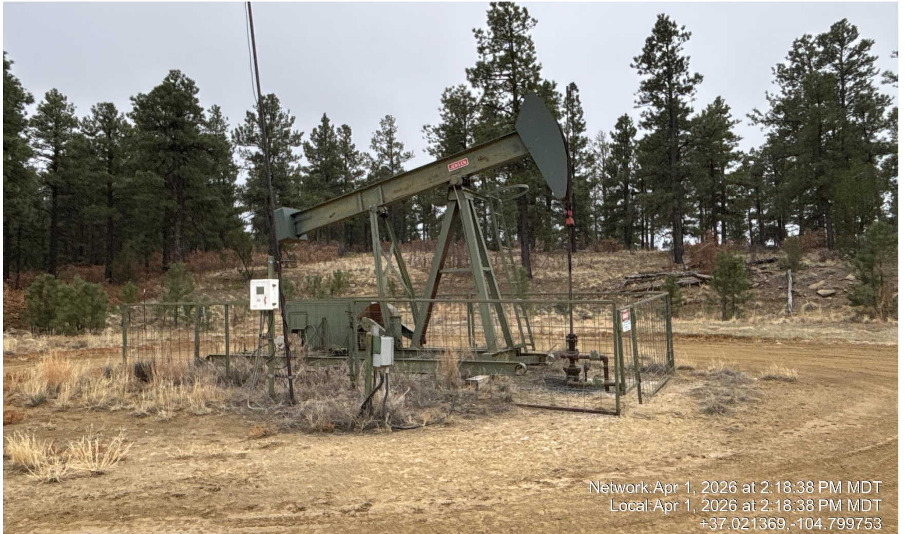
PHOTO 4: WELLHEAD AND EQUIPMENT.
