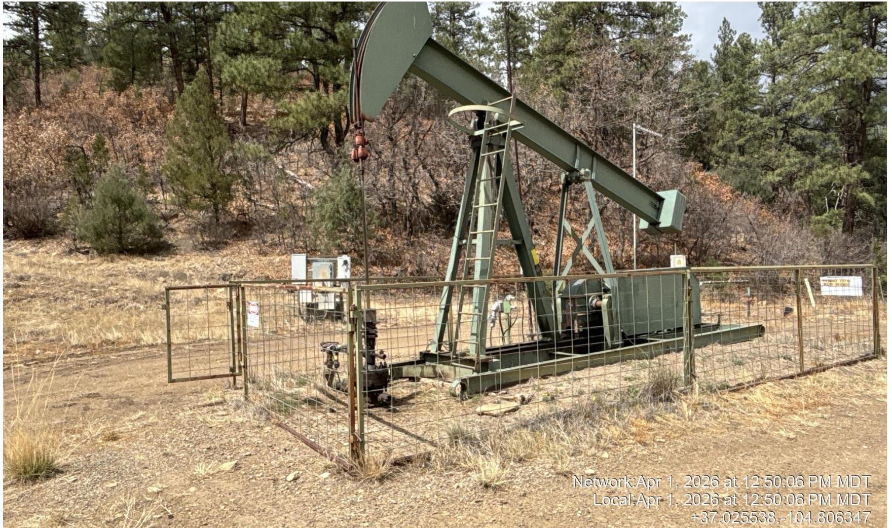
PHOTO 4: WELLHEAD AND EQUIPMENT.
