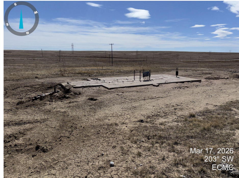
Photo 6. Looking South across the wellhead area. Pipe riser, concrete pad and electrical poles remain. Subsidence was observed around the wellbore.
