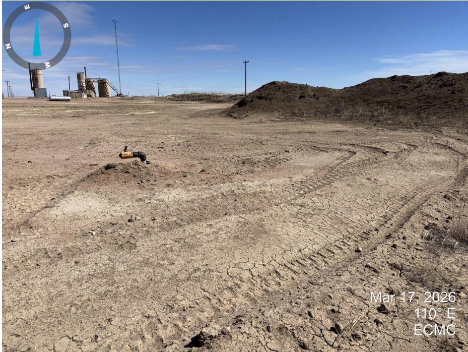
Photo 3. Looking east across the former tank battery area. Pipe riser remains on location. Contaminated soil pile does not have any stormwater BMPs surrounding it.
