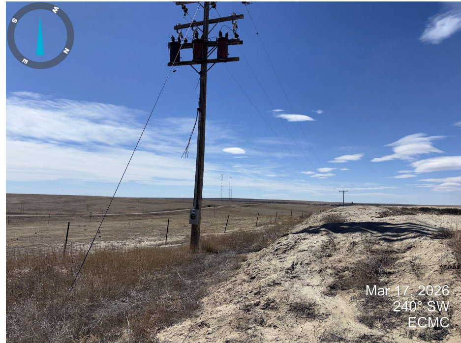
Photo 2. Electric poles terminate at the tank battery and remain in place.
