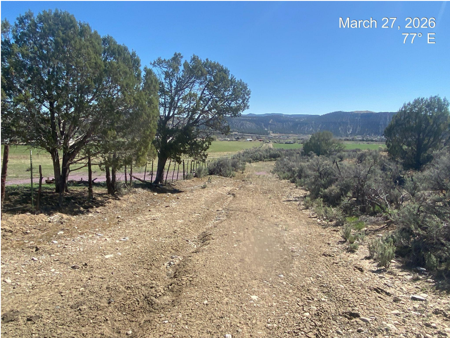
Photo 6. View of the access road. Portions of the access road has establishment of desirable vegetation. Other portions remain bare with active erosion issues.
