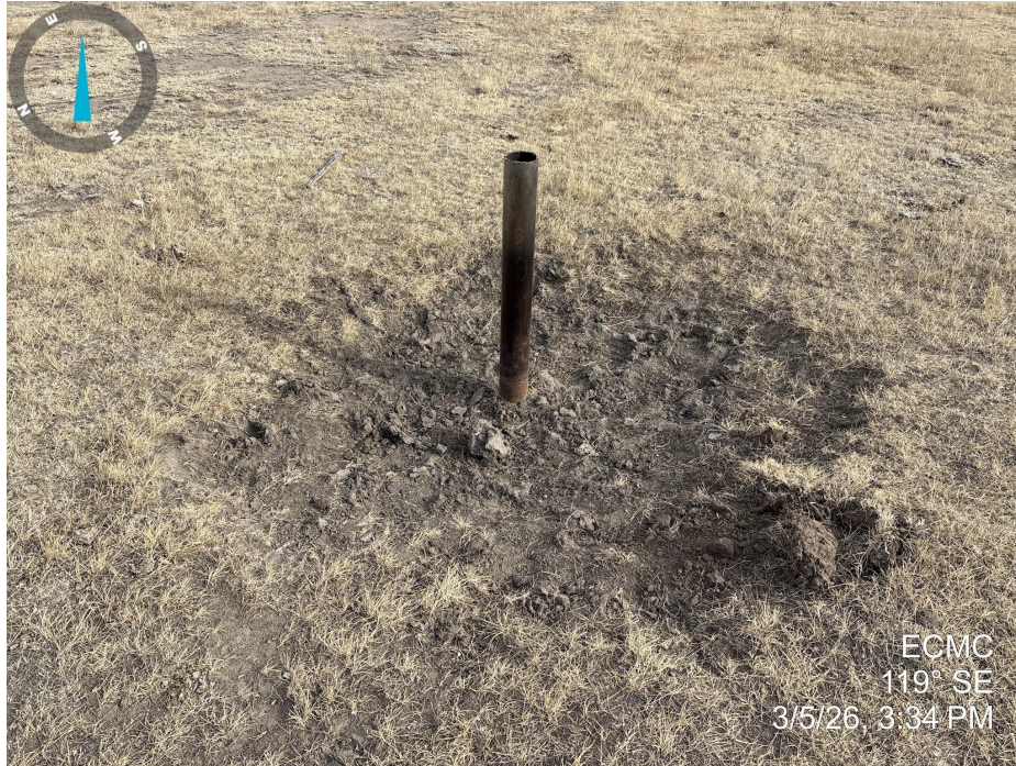
Photo 5. Photo taken of the well location, facing southeast. There is a PA marker with an unwelded cap and bare ground.
