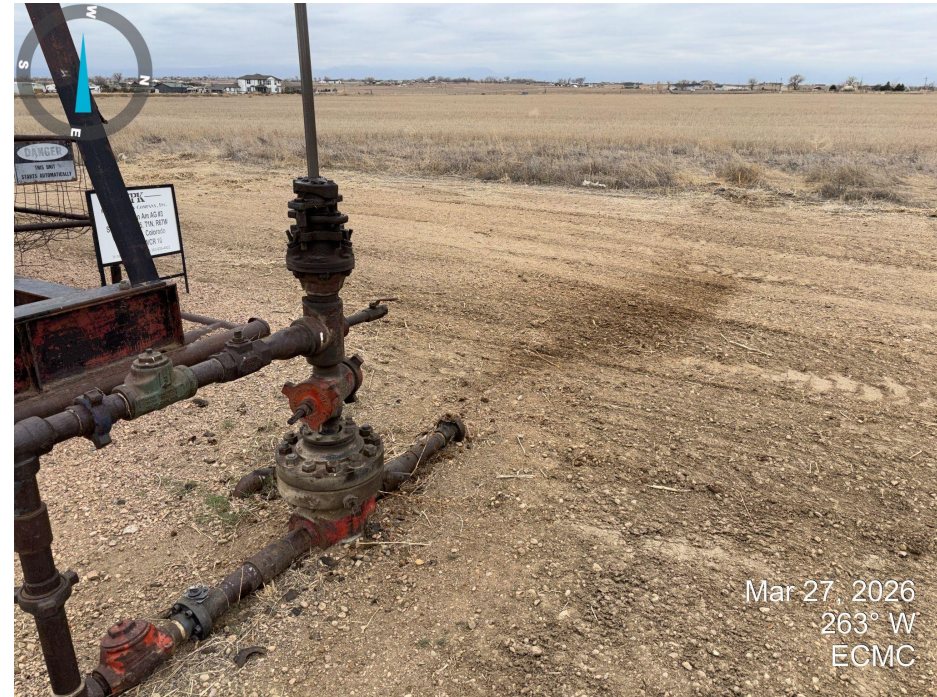
Photo 2. There appears to be stained soil to the west of the wellhead possibly blown out of the fitting near the ground.
