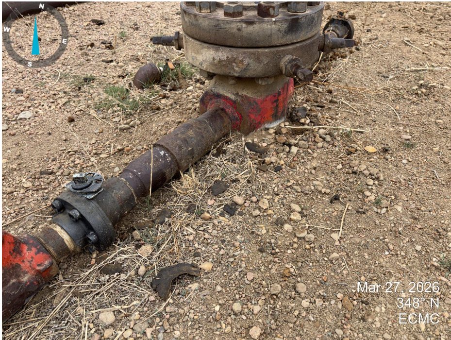
Photo 3. Solid debris also present around the wellhead.
