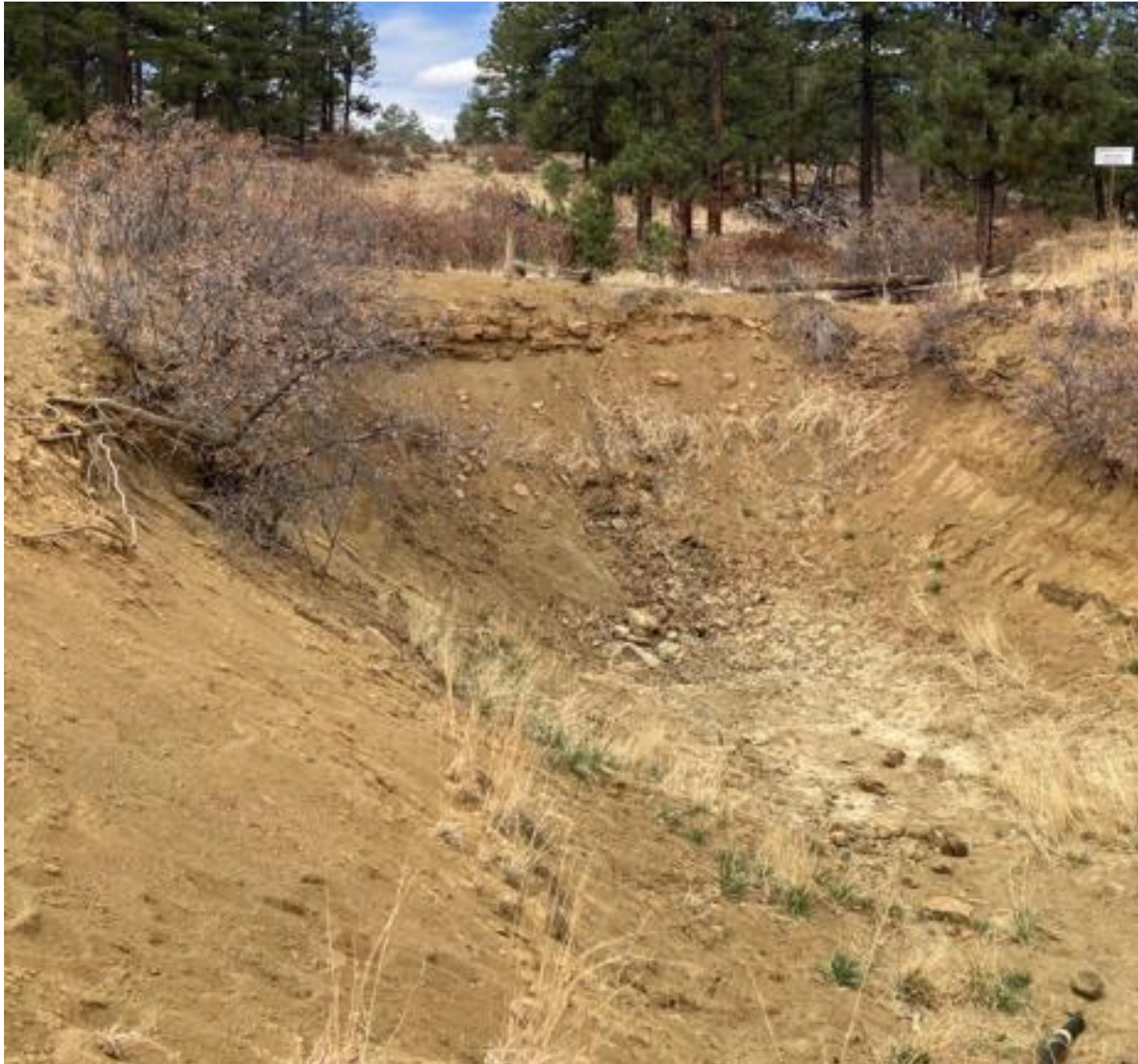
PHOTO 2: THE DEAD TREES HAVE BEEN REMOVED FROM THE PIT.
