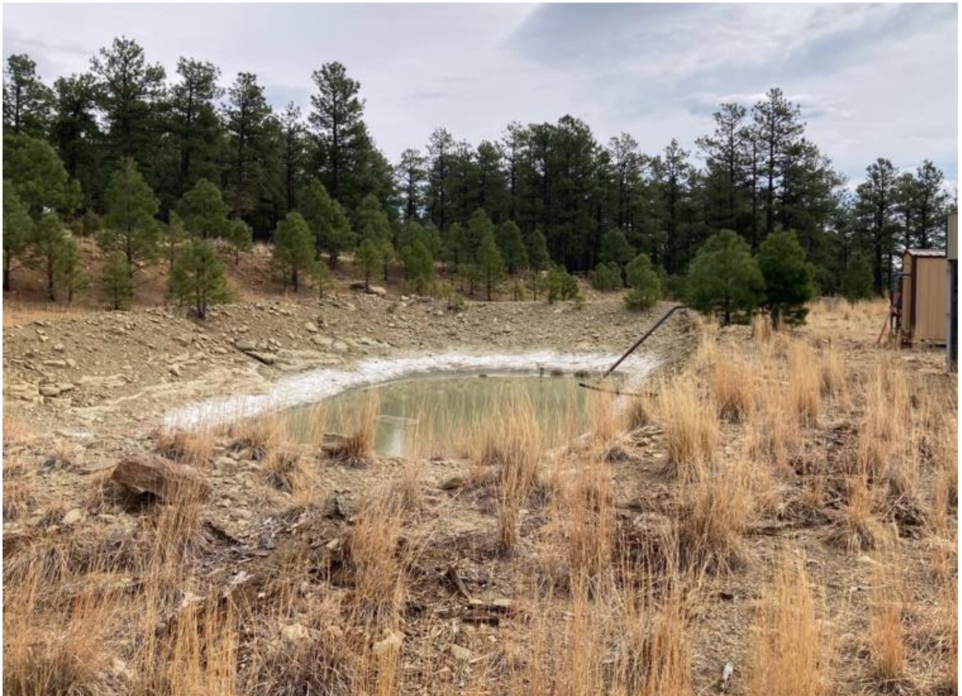
PHOTO 2: THE PIT FENCE HAS BEEN REMOVED.
