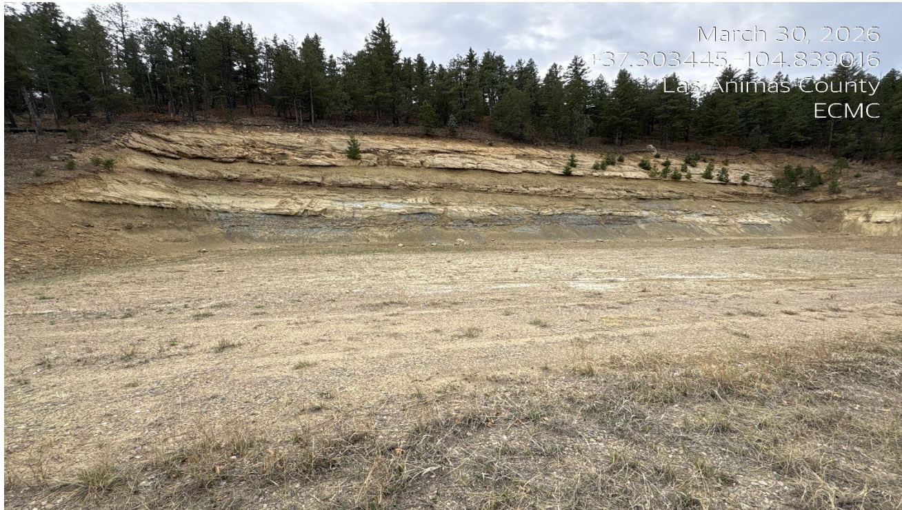
Photo 1. Facing south at the location. The location has not been recontoured and a steep cut slope remains. Previous corrective action not completed. .
