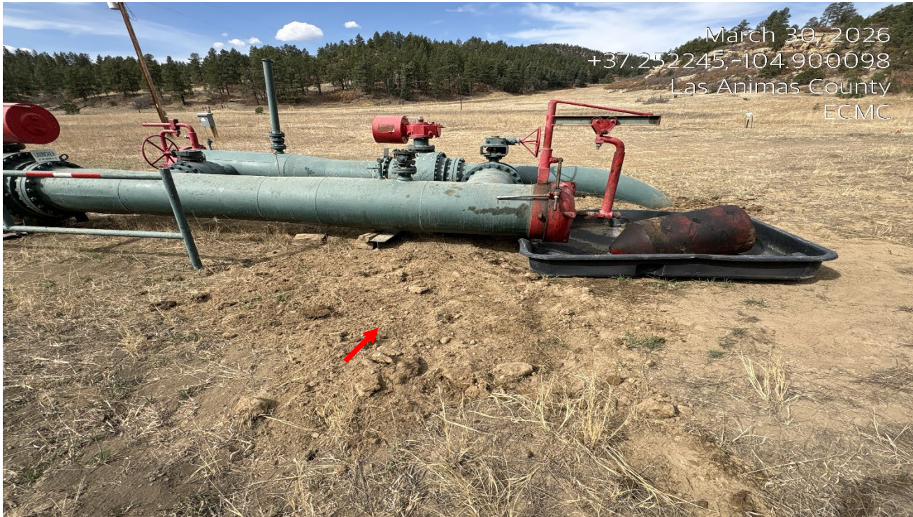
Photo 3. There is impacted material shown at red arrows that needs to be cleaned up.
