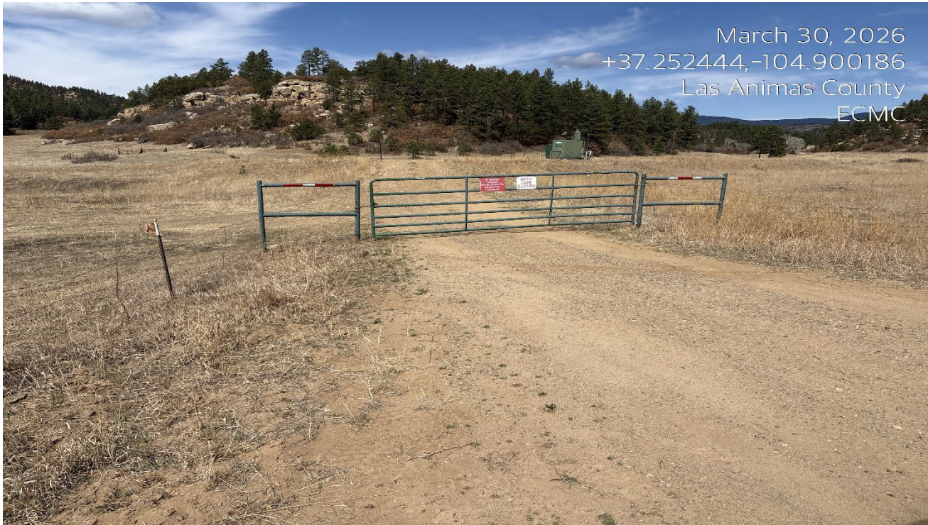
Photo 1. Facing northwest at the access road. The gate has been repaired.
