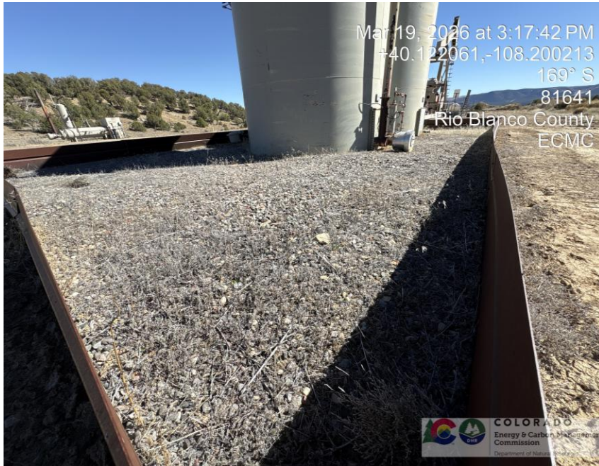
Photo # 3470 Dead weeds/debris
