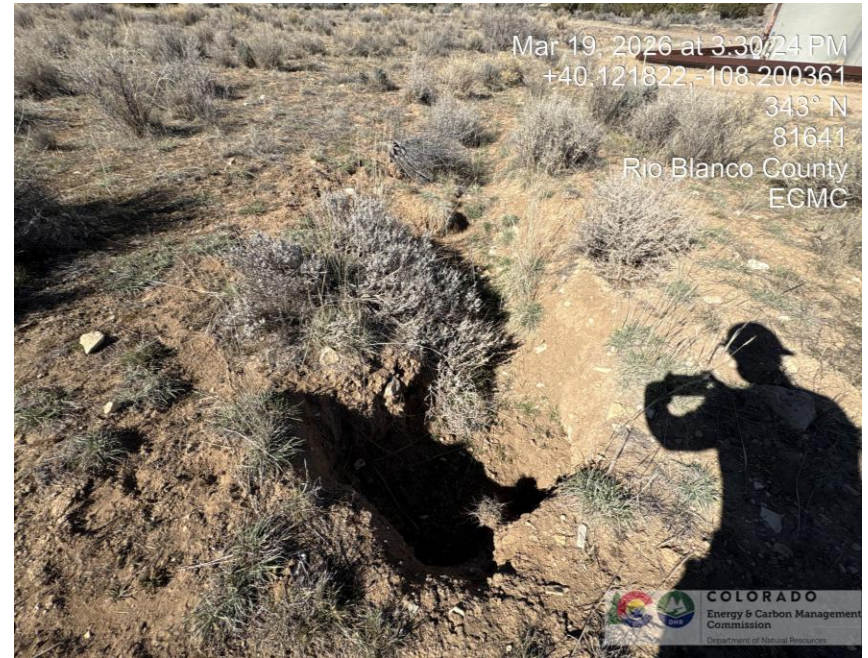
Photo # 3487 Subsidence on west side of location
