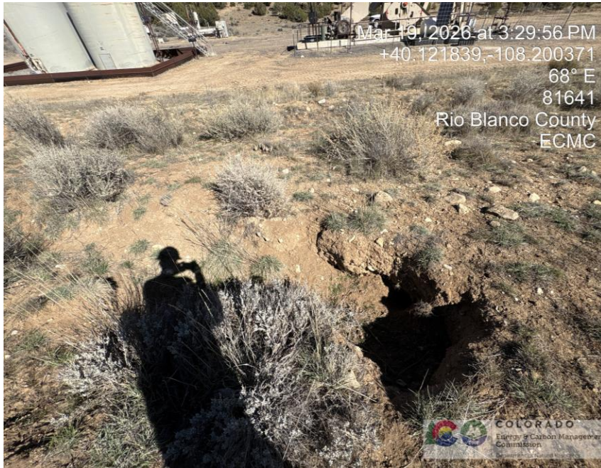
Photo # 3485 Subsidence on west side of location
