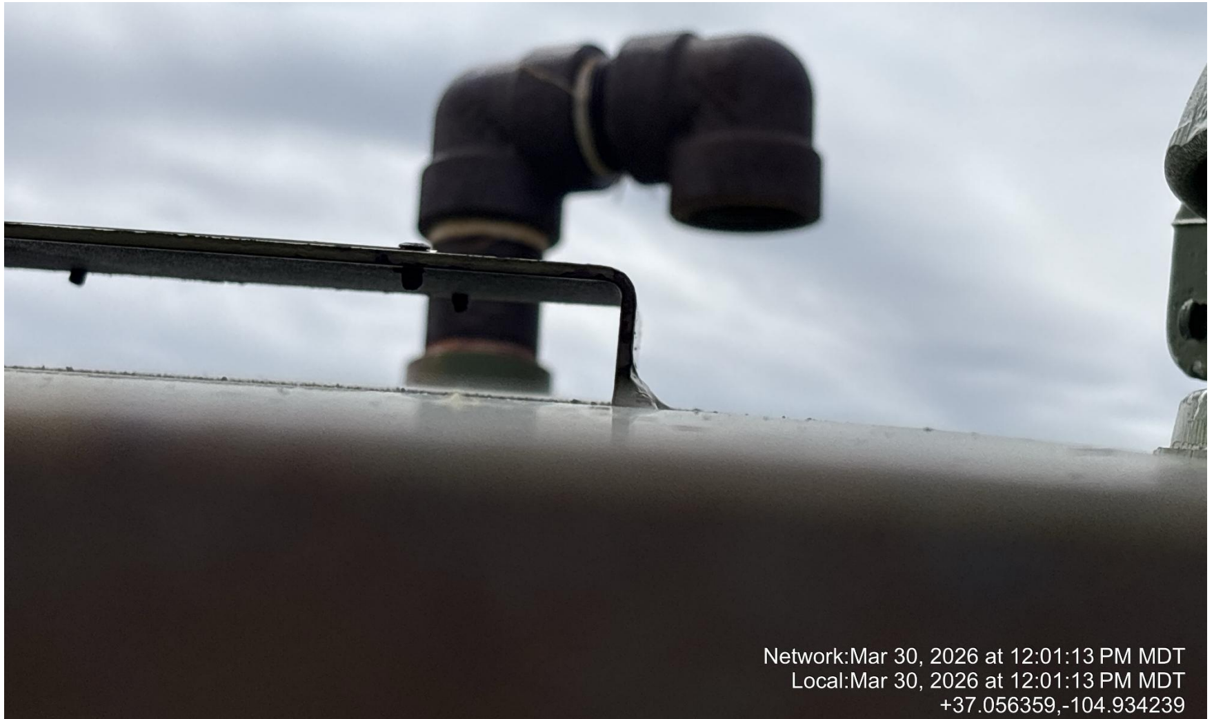
PHOTO 4: NEED TO ADD WILDLIFE PROTECTION ON 25 BBL PRODUCED WATER TANK.
