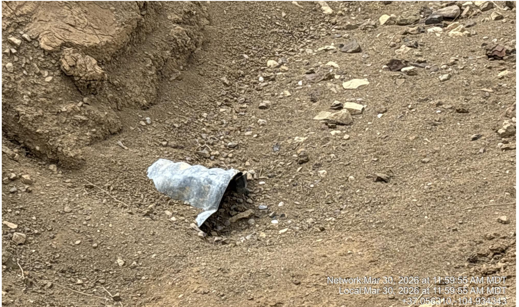
PHOTO 5: CULVERT NEEDS CLEANED. CLEAN CULVERT PER RULE 1002. CA DATE 4/15/2026.
