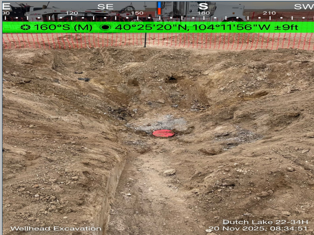
View of overall wellhead excavation
