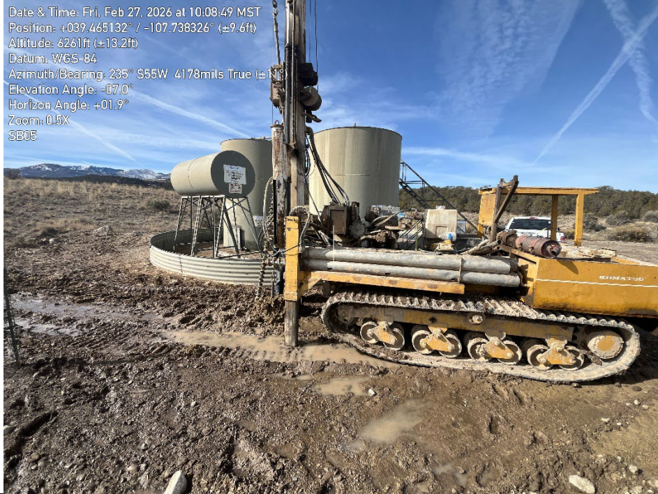
View facing southwest of soil boring SB05.
