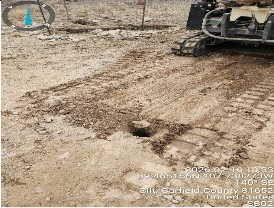
View facing southeast of soil boring SB02.
