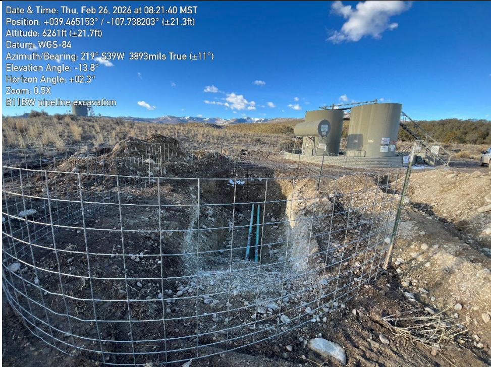
View facing southwest of the pipeline excavation.
