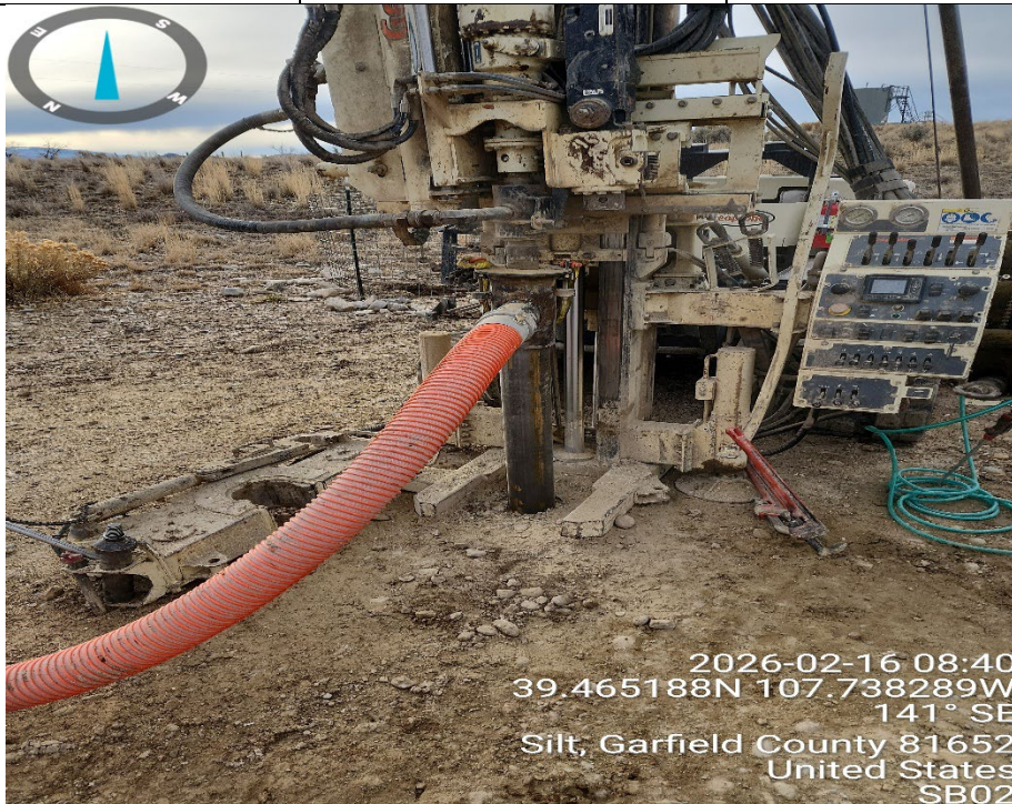
View facing southeast of soil boring SB02.
