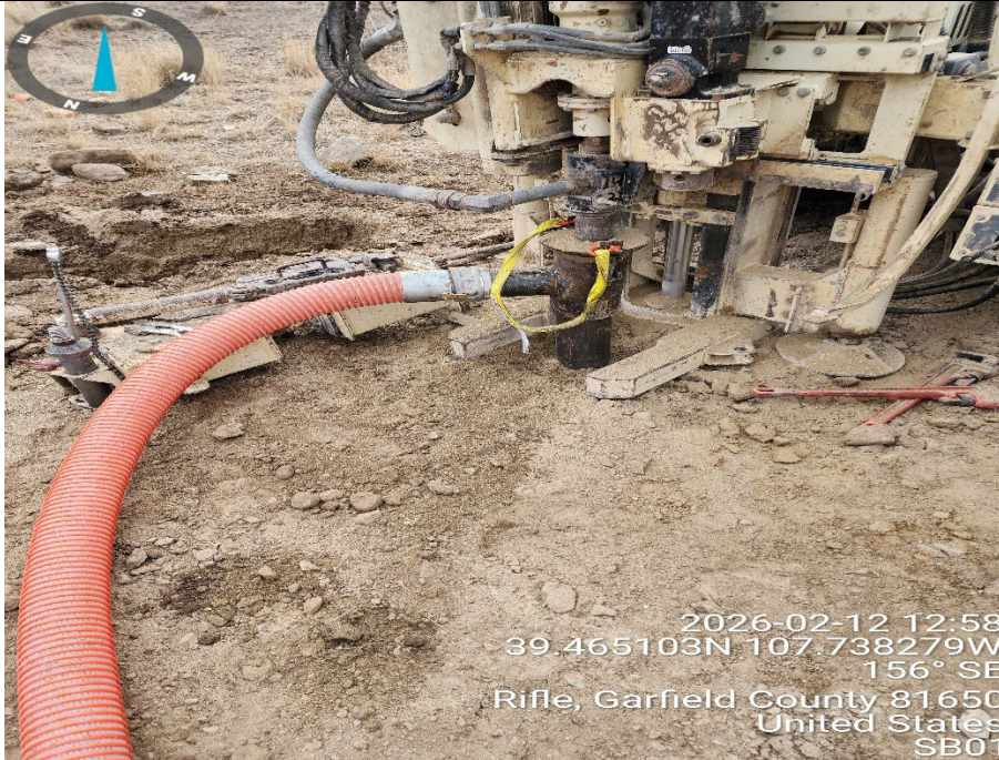
View facing southeast of soil boring SB01.
