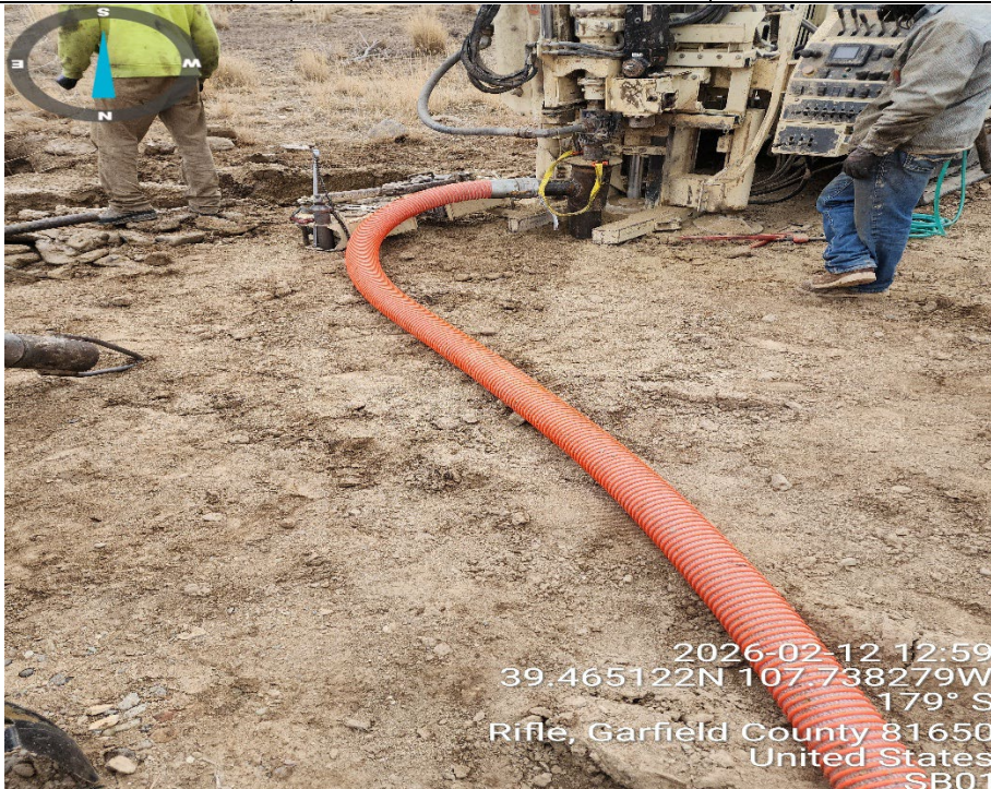
View facing southeast of soil boring SB01.
