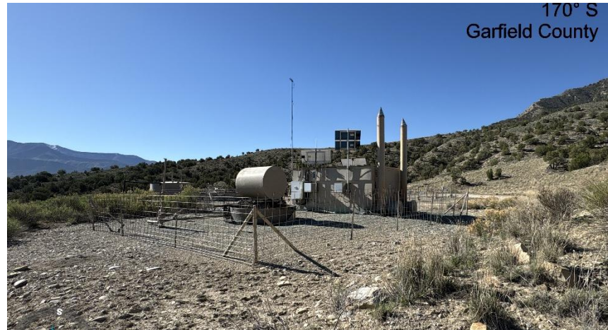
North East corner of location.
