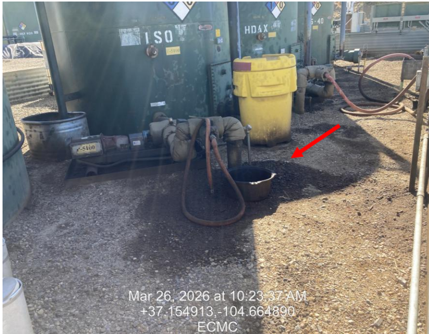
Photo 9: TB # 2 upper level , impacted soils
