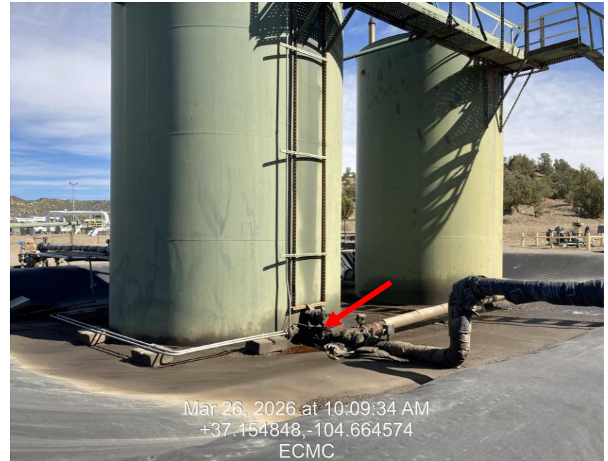
Photo 4: TB # 1 Upper Level, oily residue, free product/oily mix
