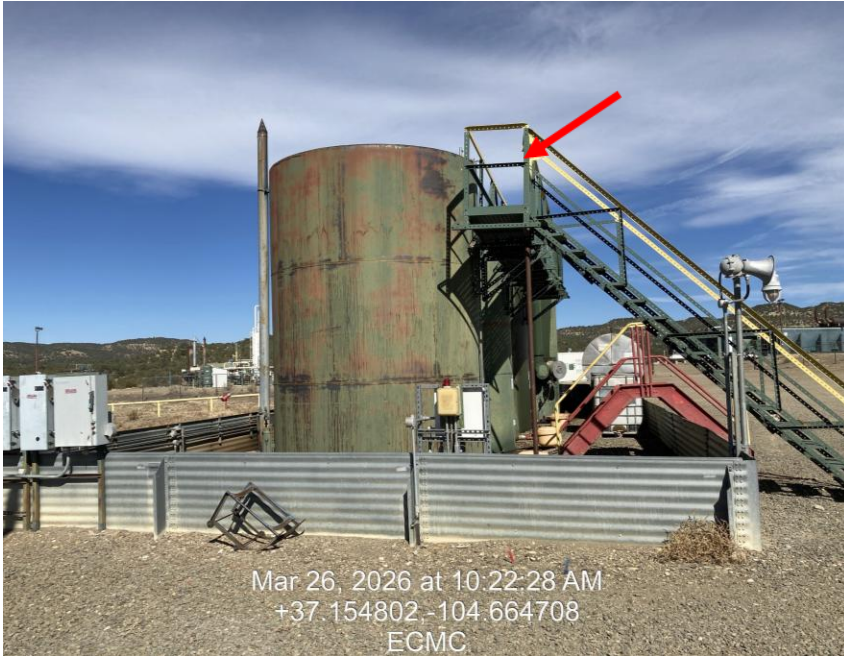
Photo 5: TB # 2 upper level
