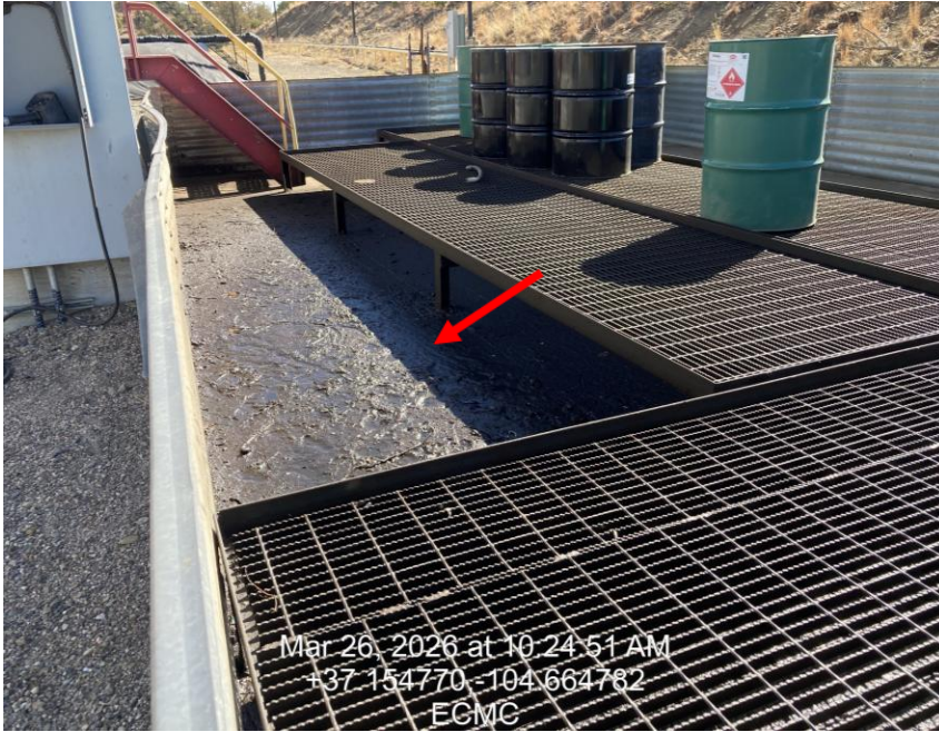
Photo 11: Containment upper level, oily residue on cement floor
