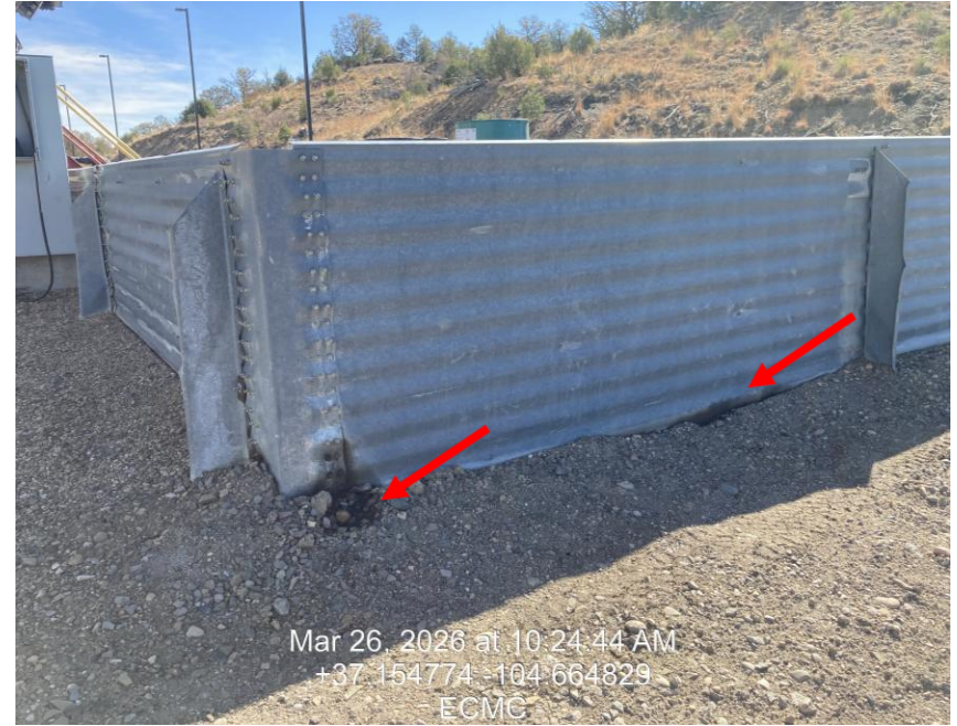
Photo 12: Containment upper level, oil-stained soils outside containment
