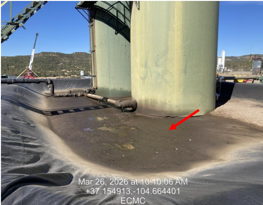
Photo 3: TB # 1 Upper Level , oily residue in containment
