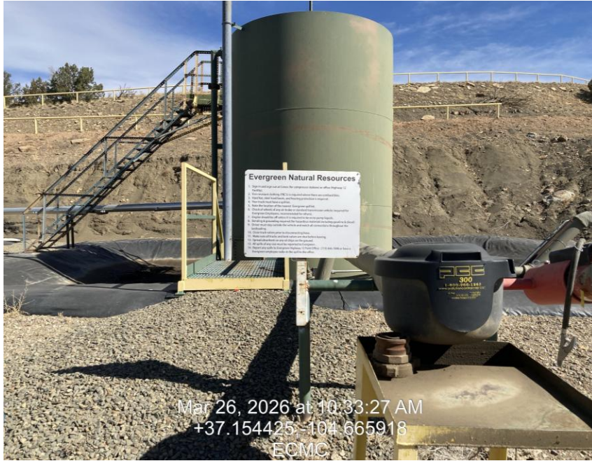
Photo 16: TB # 1 Lower Level,
