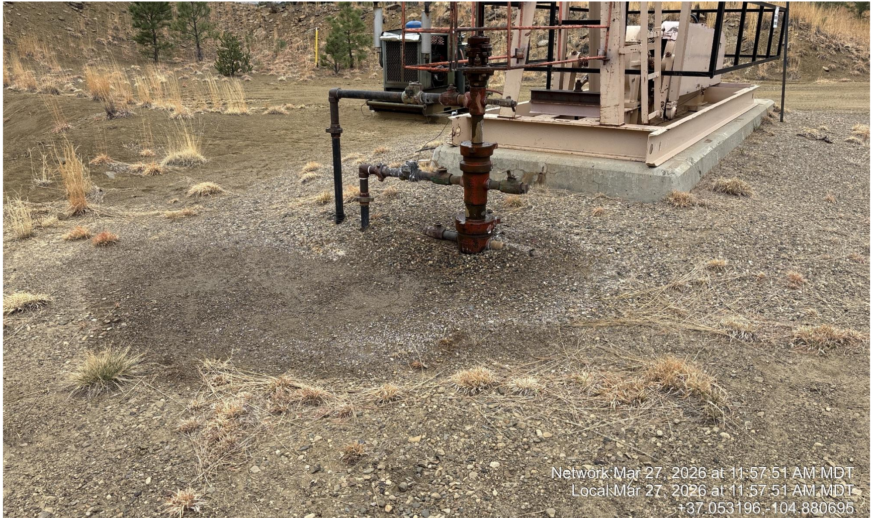
PHOTO 7: ALLTHOUGH IT APPEARS THAT THE CA FROM PREVIOUS INSPECTION WAS ADDRESSED THE CONDITIONS THAT CREATED THE CA STILL EXISTSON V WELL. Securely fasten all valves, pipes, fittings, and Production Facilities to ensure good mechanical condition, inspect at regular intervals and maintain in good mechanical condition. Engineer, operate, and maintain equipment within the manufacturer’s recommended specifications per Rule 608.e. CA DATE 4/2/2026.
