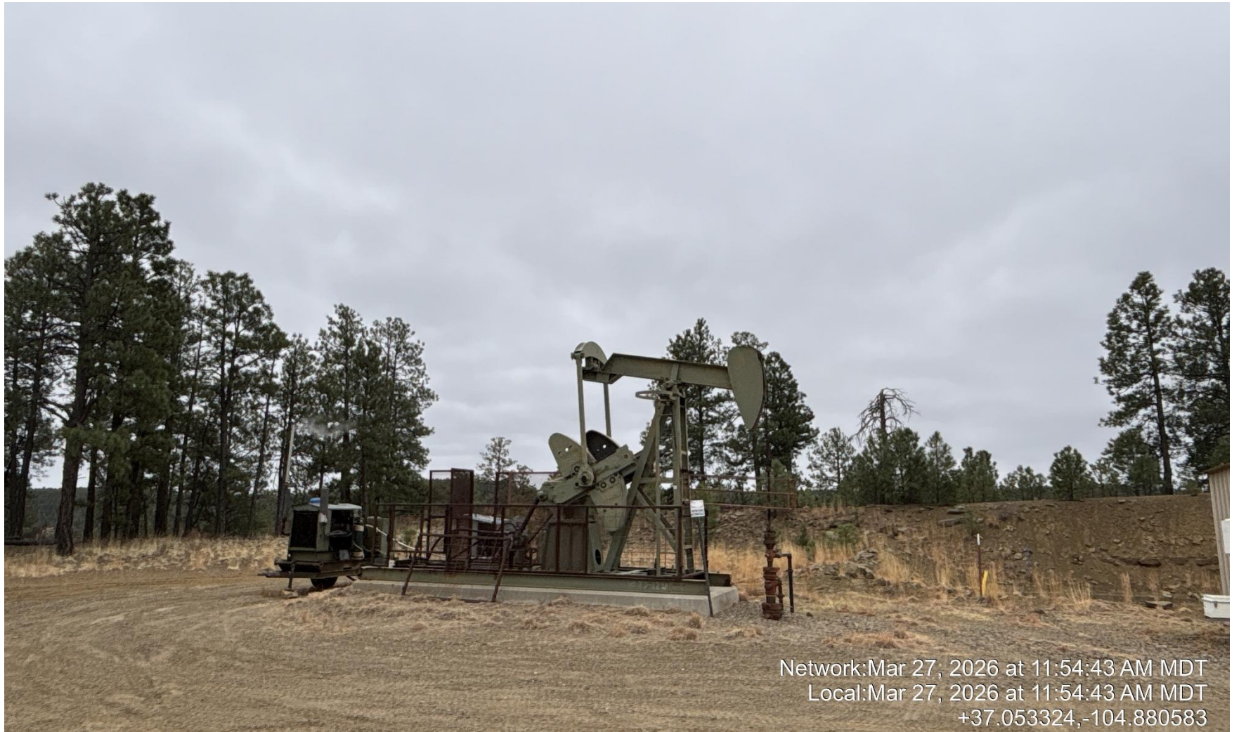
PHOTO 4: R WELLHEAD AND EQUIPMENT.
