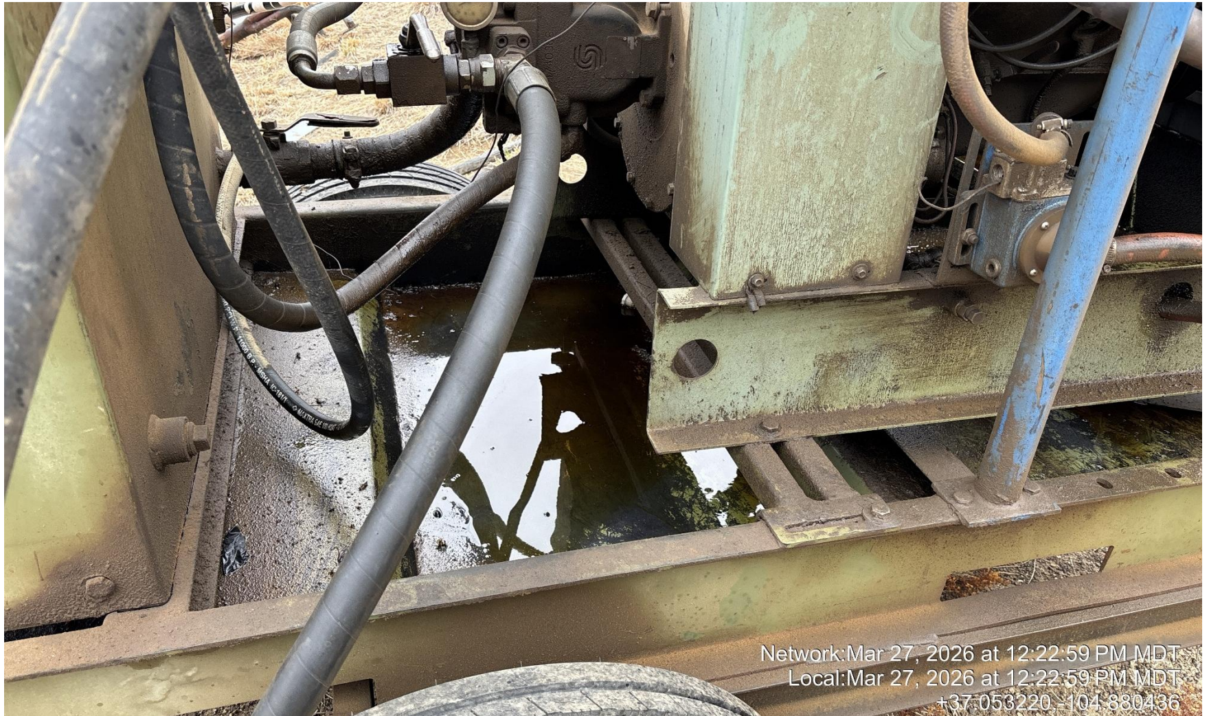
PHOTO 8: OILY WASTE IN PRIME MOVER ENGINE SKIDWITHOUT WILDLIFE PROTECTIONS ON R WELL. DRAIN OILY WASTE REPAIR ALL LEAKS AND REMOVE IMPACTED SOIL PER RULE 1002..(2).D & 1002.f.(2)B, Comply with general provisions of the oil and gas act for wildlife protection AND SB-181. CA DATE 3/28/2026.
