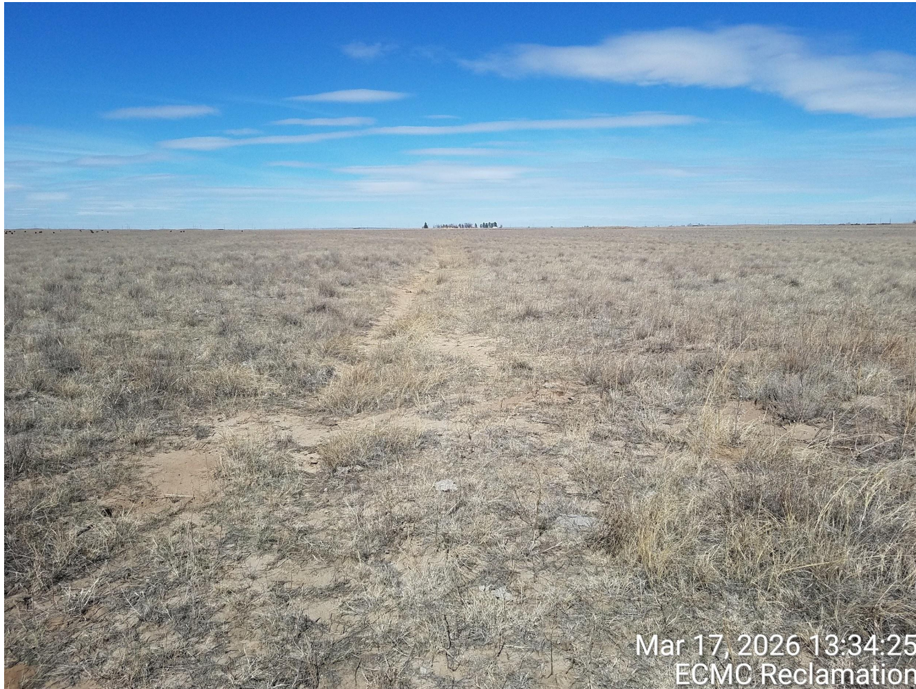
Photo 7. Photo taken from the well location, facing North. Photo illustrates the access road vegetation meets Rule 1004 standards with the establishment of perennial, native grasses.
