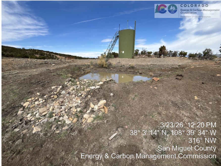
Retention pond on SE corner of tank battery
