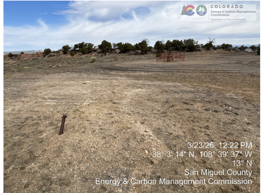
Unmarked guy line anchor on SW corner
