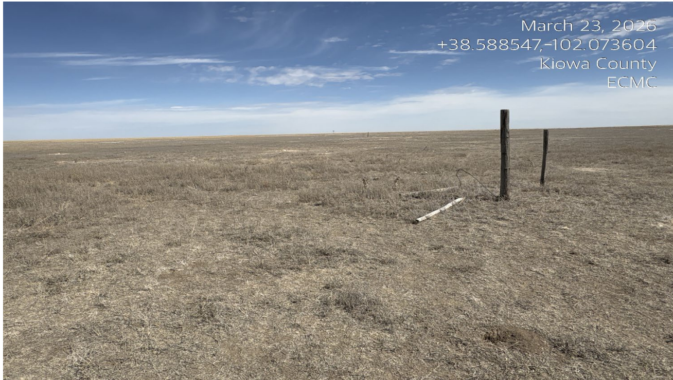
Photo 1. Facing northeast toward the location. The four corner post remain and need to be removed.
