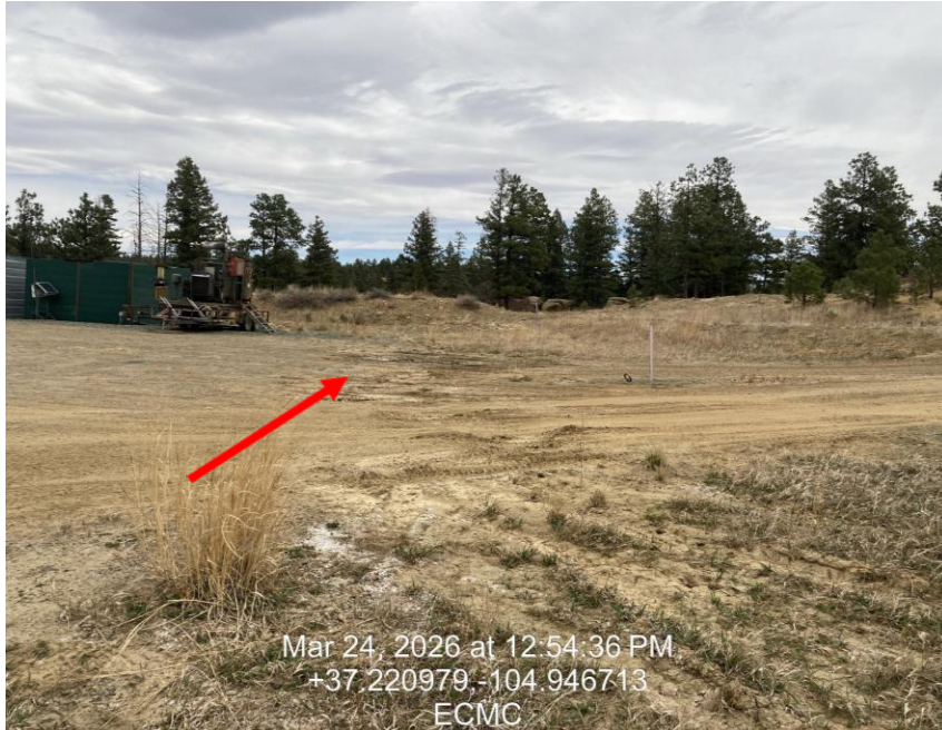
Photo 7: spill path crossing access road
