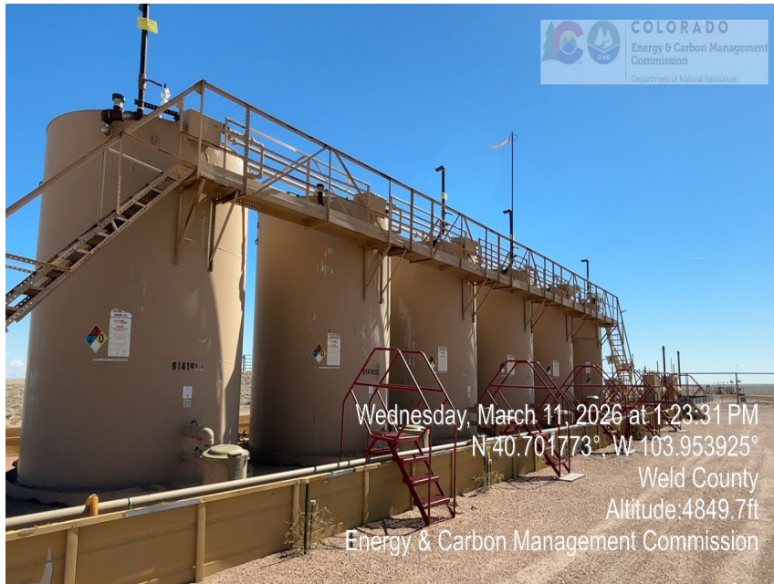
Photo 13 – Tank Battery
