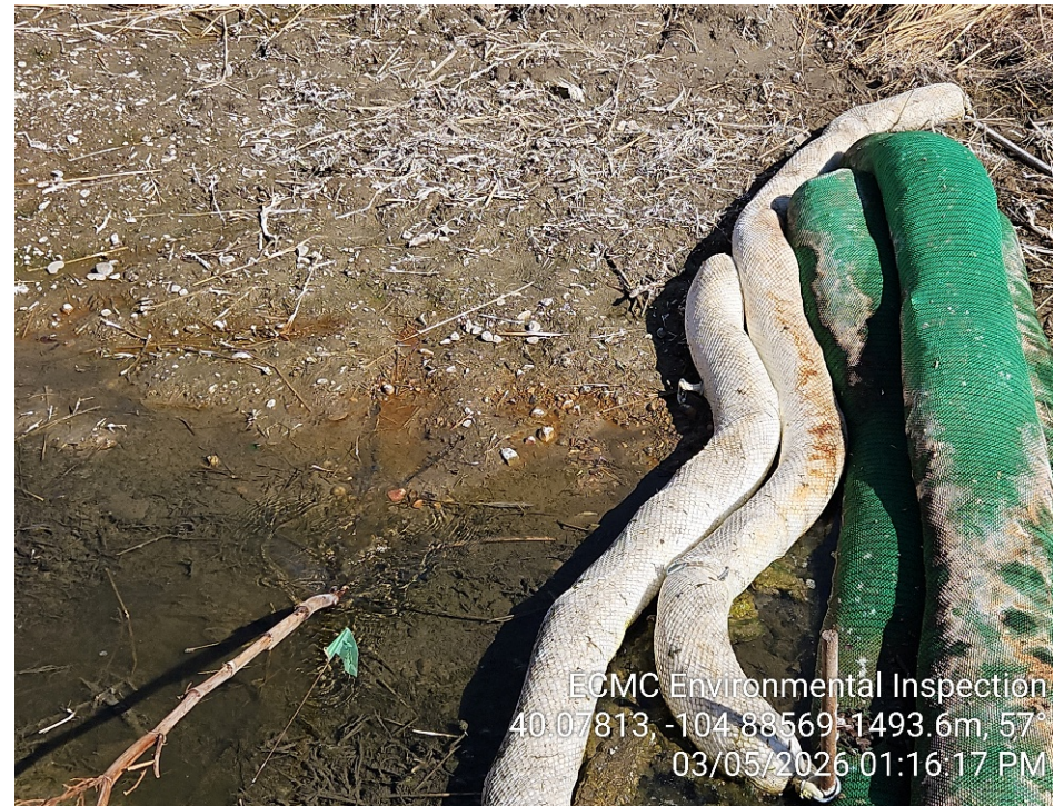
Photo 10 – Hydrocarbon sheet observed when soils in Big Dry Creek were disturbed.
