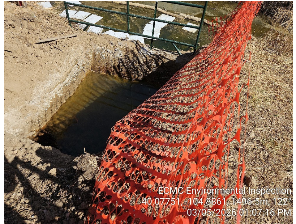
Photo 2 – Small excavation on location. Impacts present in sidewall and free product on groundwater.
