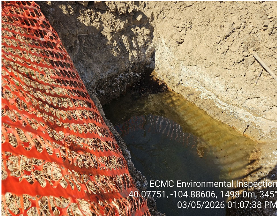
Photo 1 – Small excavation on location. Impacts present in sidewall and free product on groundwater.
