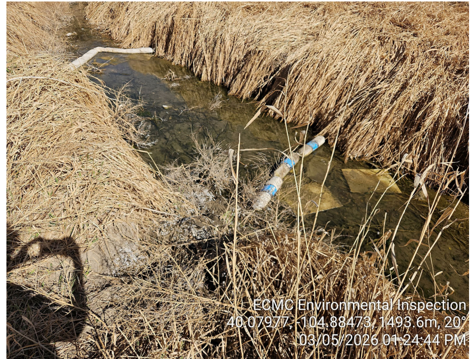
Photo 12 – Booms and mats placed in Big Dry Creek have not been maintained and require replacement.
