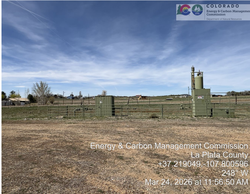
7. Meter run and vertical heated separator.
