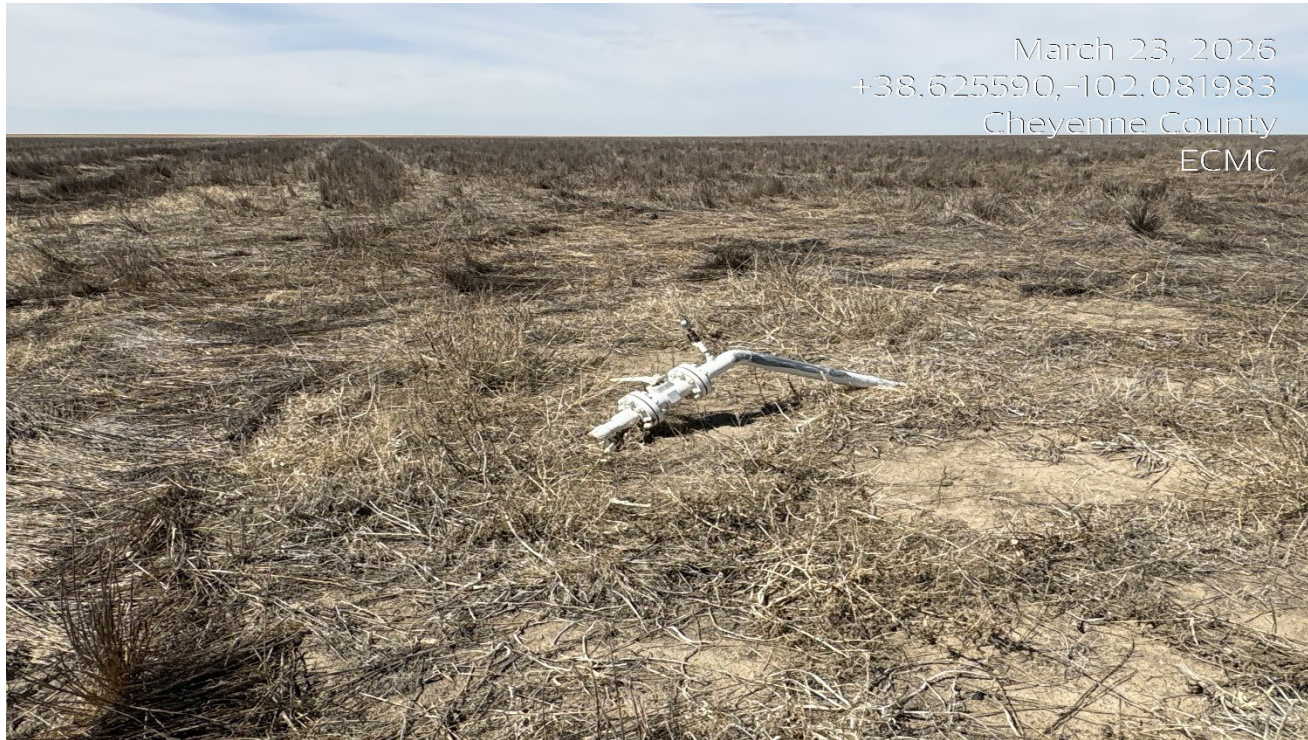
Photo 1. Facing west at the location. There is a pipe riser that needs to be removed. The riser is low to the ground and could be a farming hazard.
