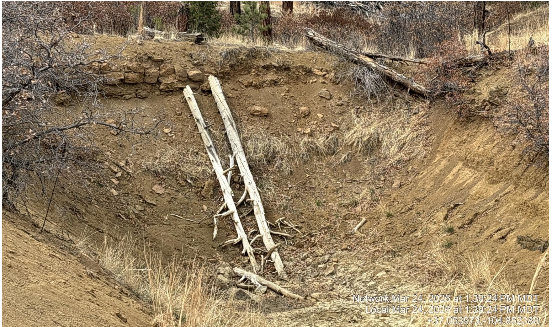
PHOTO 6: DEAD TREES AND DEBRIS INSIDE AND ON BANK OF PRODUCED WATER PIT. REMOVE TREES AND DEBRIS PER RULE 606. CA DATE 3/30/2026
