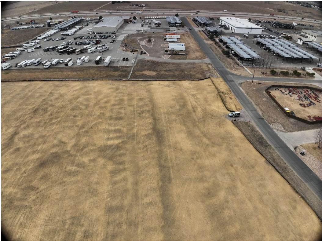
In View – Tank Battery, Flowlines
