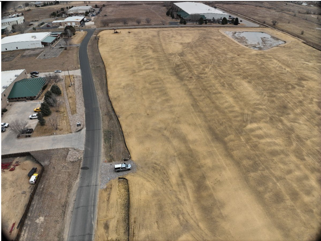
In View – Wells, Tank Battery, Flowlines
