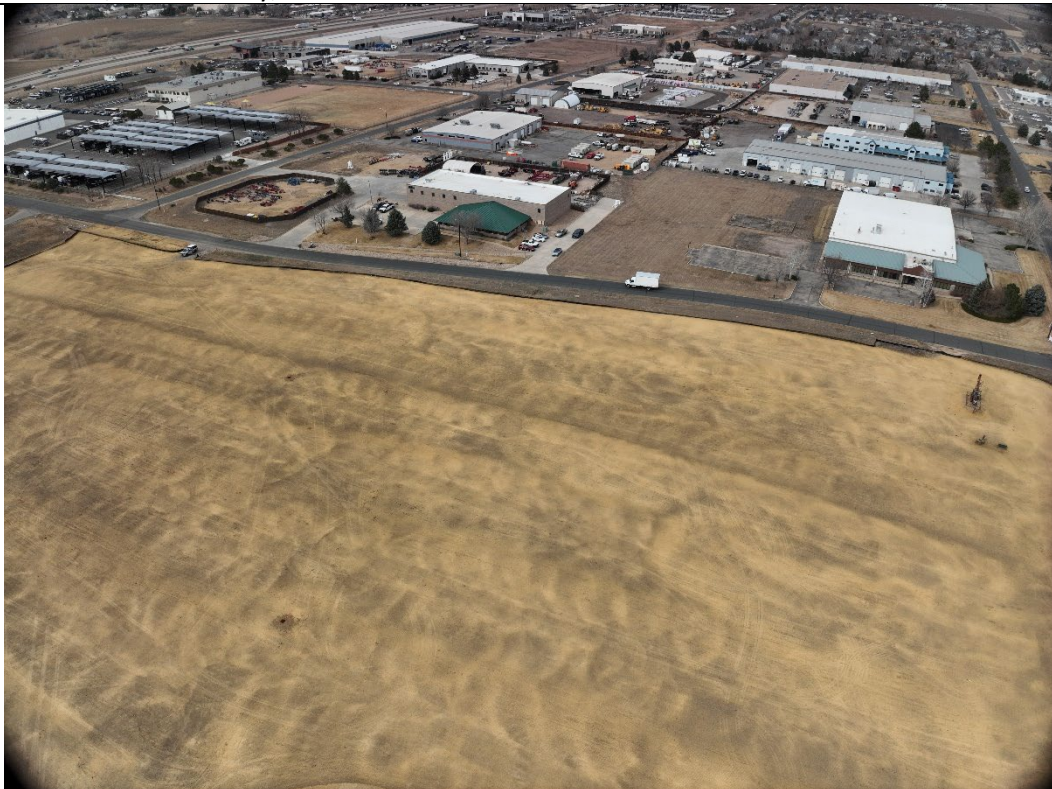
In View – Wells, Tank Battery, Flowlines
