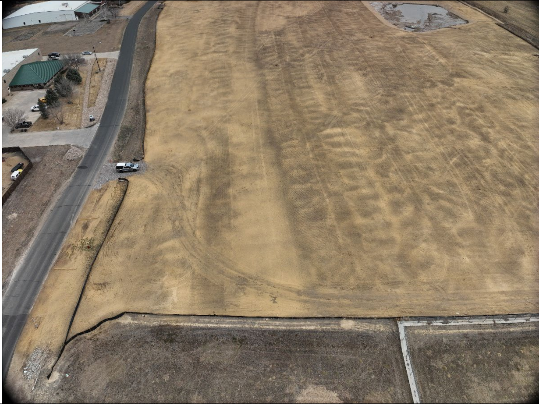
In View – Tank Battery, Flowlines
