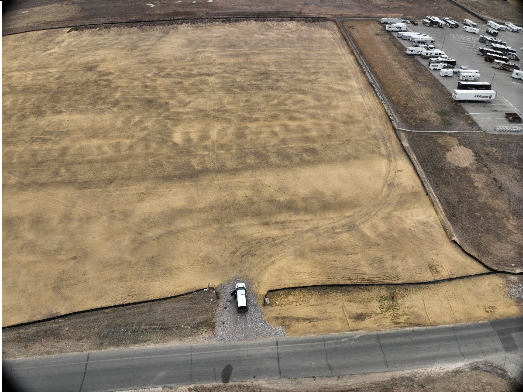
In View – Tank Battery, Flowlines
