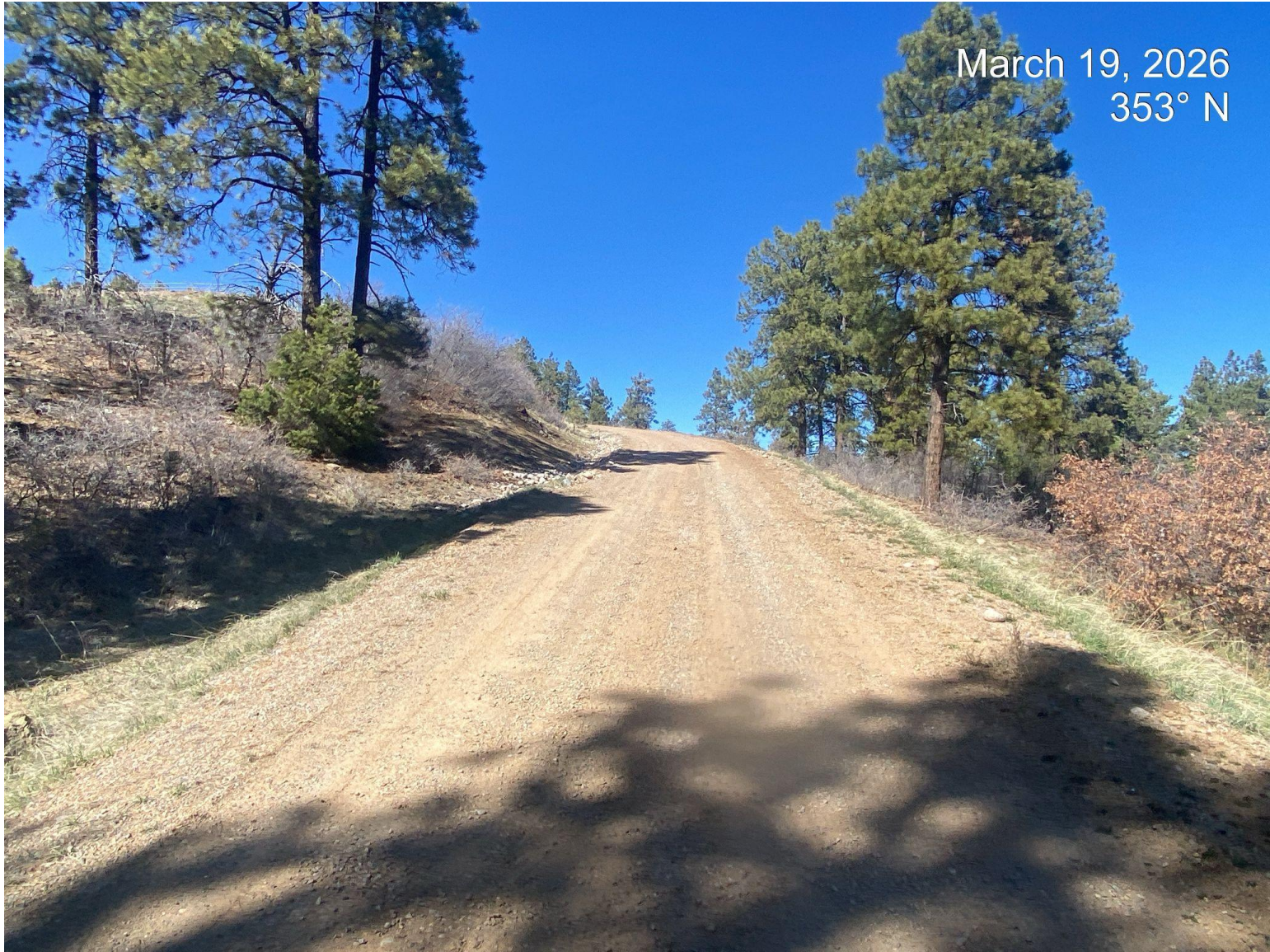
Photo 2. View of location access road, no stormwater issues were observed.
