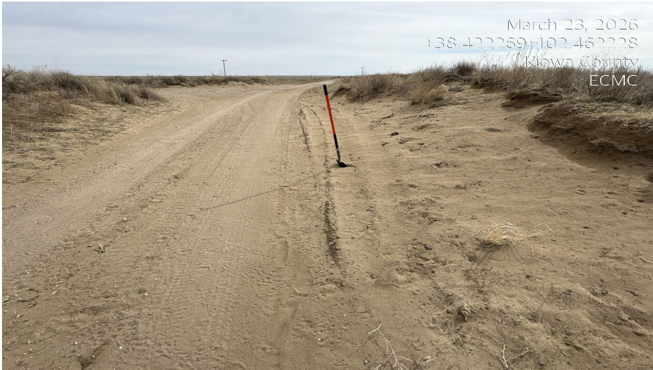
Photo 3. The roadside has eroded and is not stabilized with vegetation. The sandy soils are susceptible to further erosion. This area needs to be repaired and stabilized.
