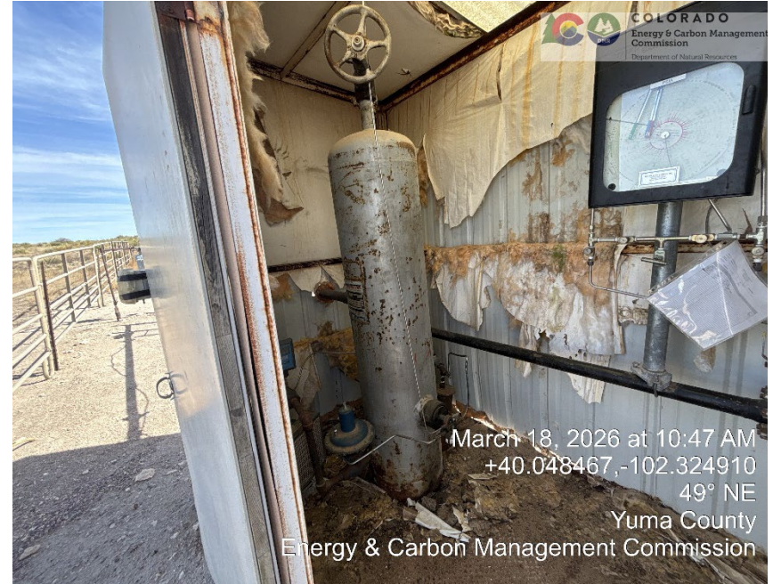
VGS and Meter
