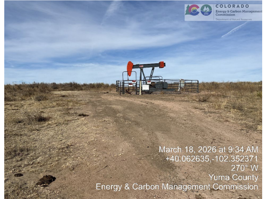
Dirt work at well
