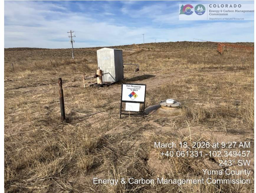
Off location shed and Tank
