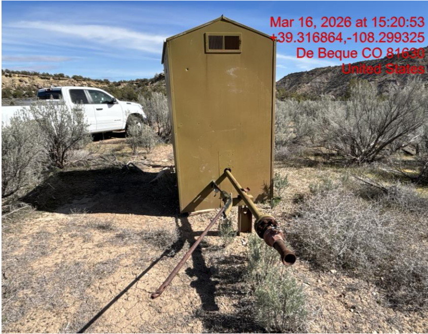
Location/Unused Equipment/Weeds – Photo #03125
