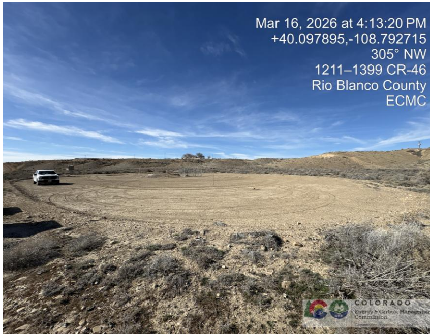
Photo # 3204 SE corner of location
