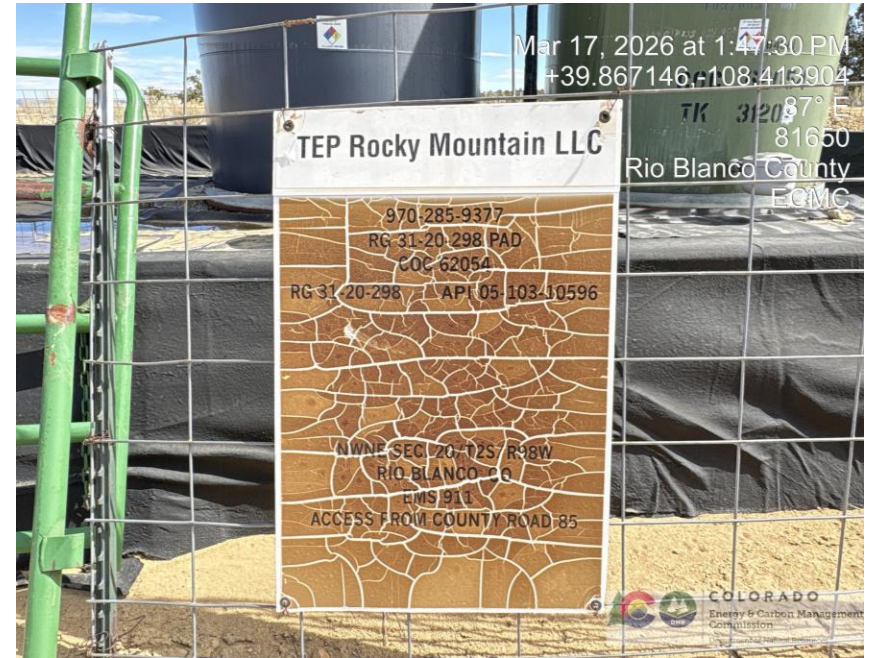
Photo # 3252 Battery sign is weathered & cracking/starting to become illegible
