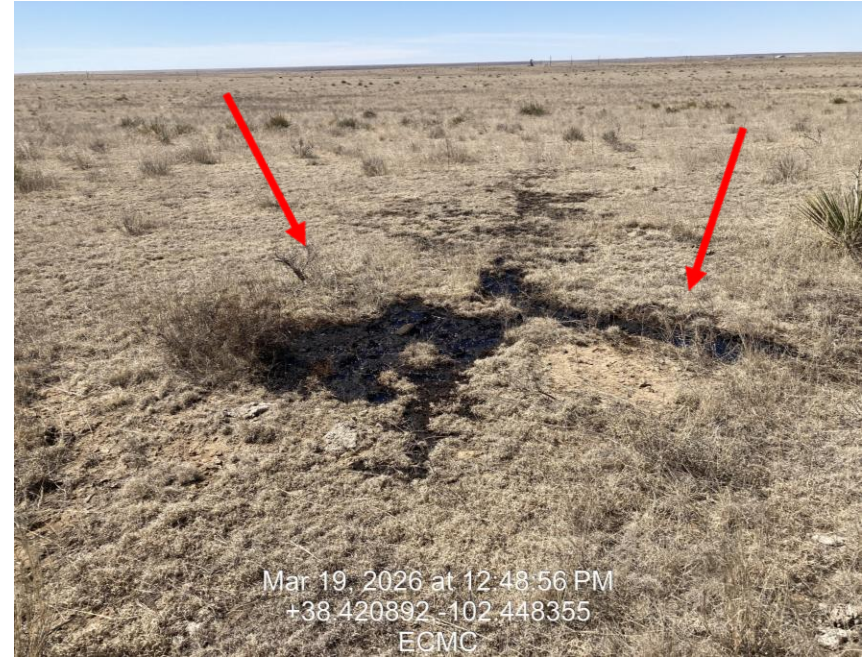
Photo 4: Oil observed along flowline
