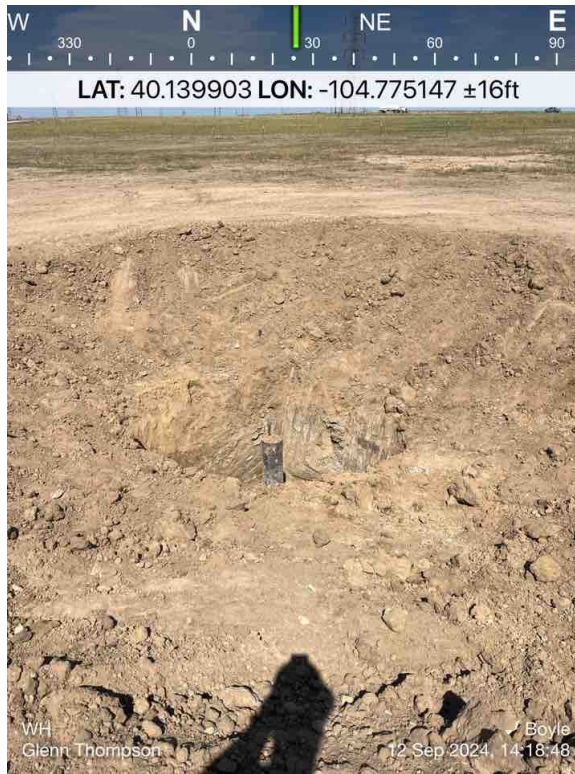
Wellhead excavation
