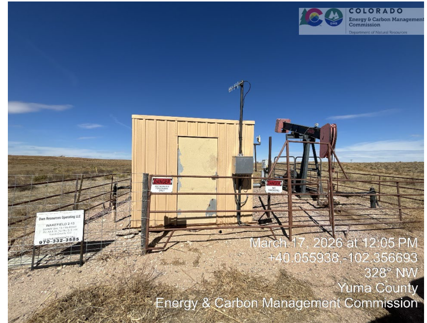
Meter run, Wellhead, and PU
