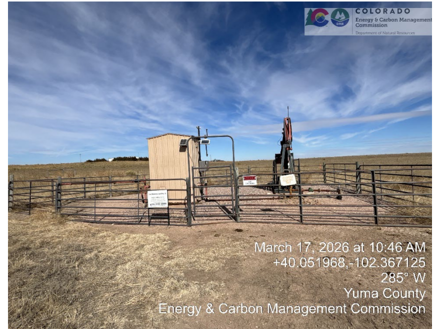
Meter run, PU, and Wellhead
