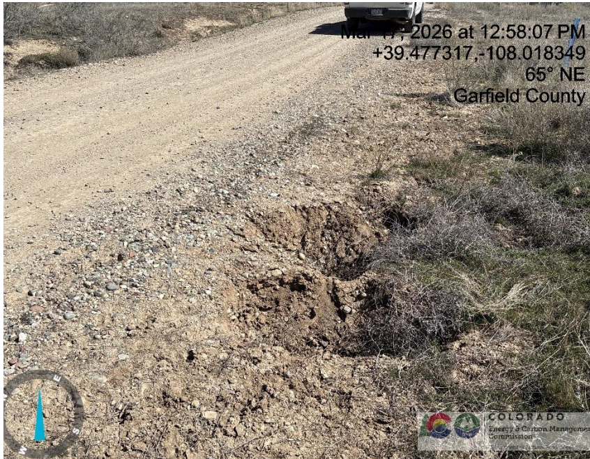
Photo # 9993 Subsidence developing along edge of lease road approximately 1/10th of a mile from entrance to location
