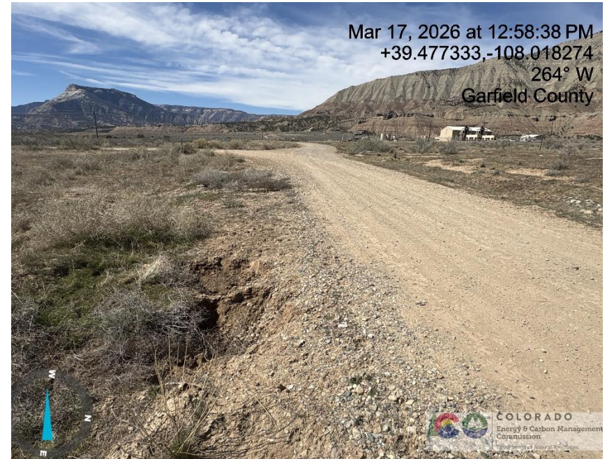
Photo # 9994 Subsidence developing along edge of lease road approximately 1/10th of a mile from entrance to location
