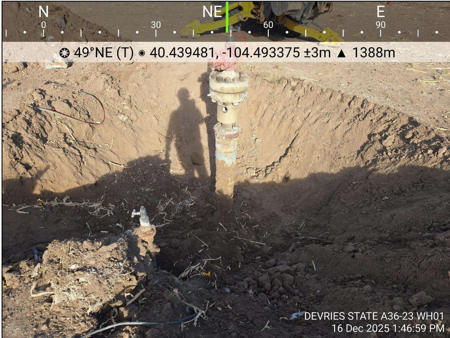
Photo 3: View of wellhead excavation extent, facing northeast
