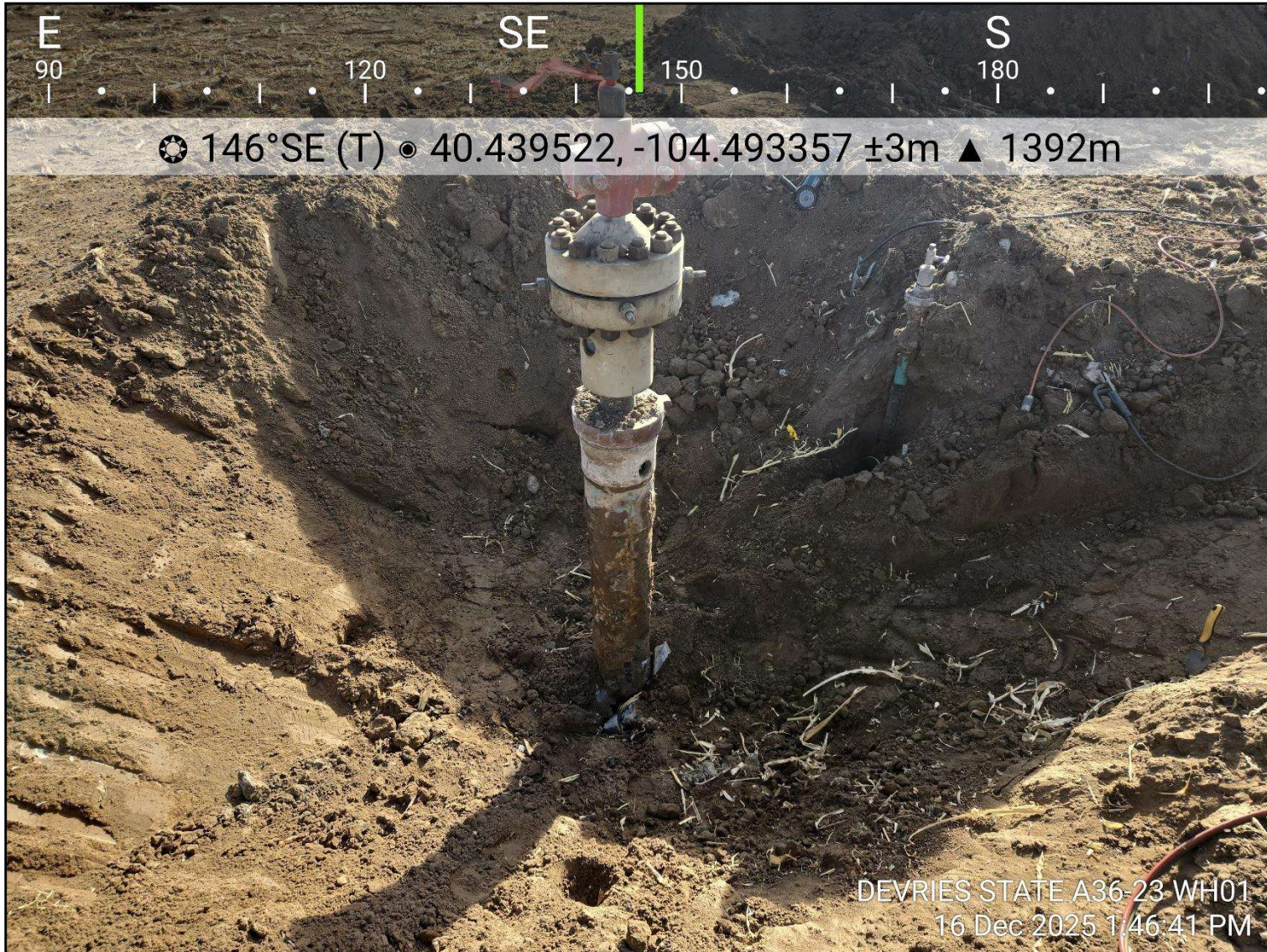
Photo 5: View of wellhead excavation extent, facing southeast
