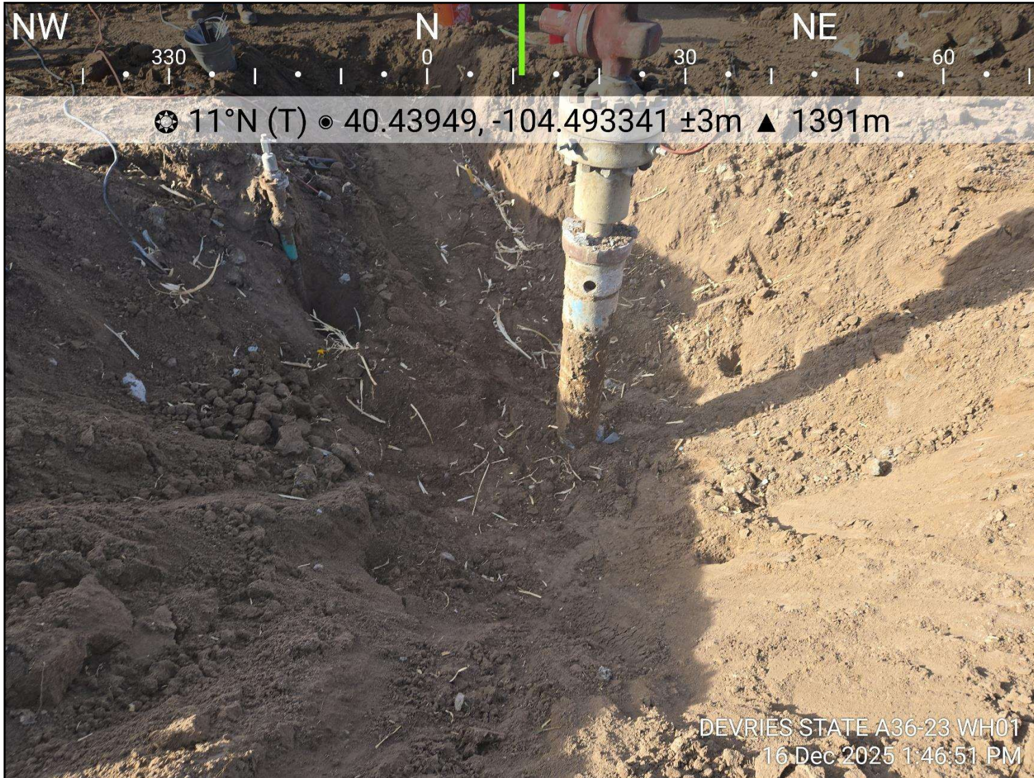
Photo 4: View of wellhead excavation extent, facing north
